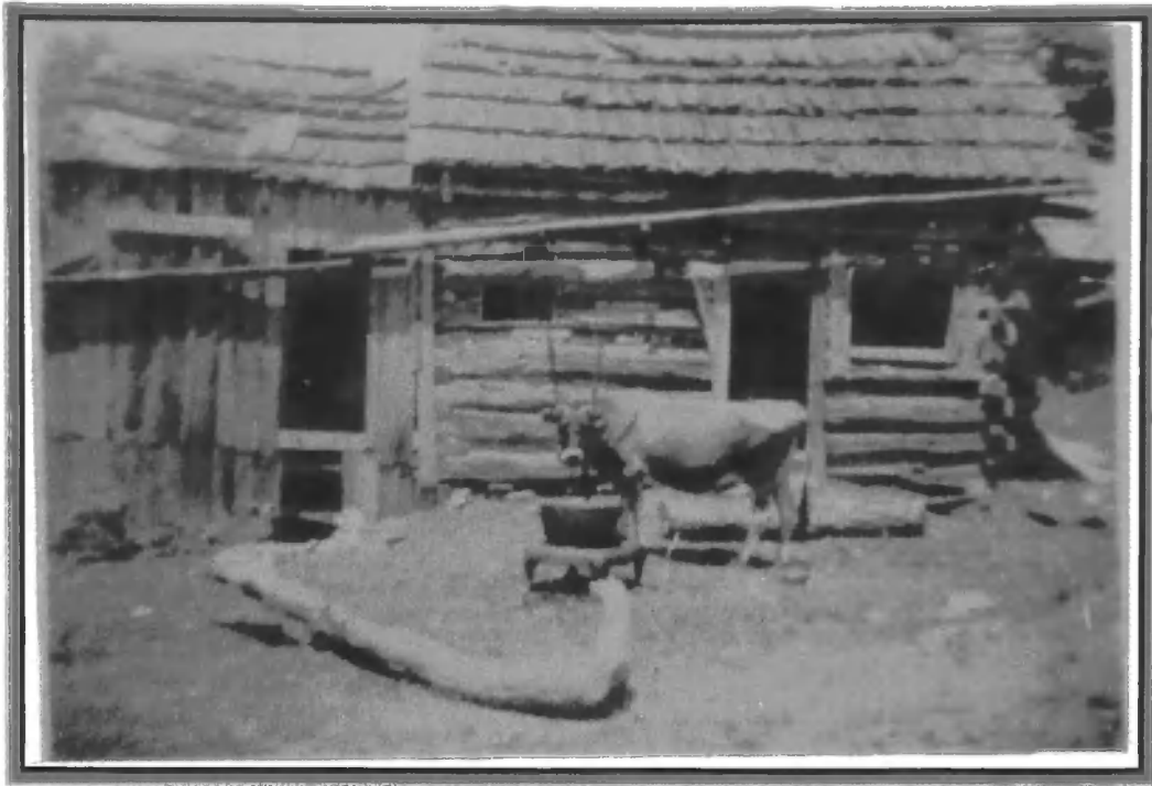
Figure 10: Thomas Gibson's log home on Chestnut Ridge. Constructed in ca. 1865.
