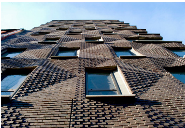
290 Mulberry uses two different brick sizes with a variable arrangement to create a contemporary facade.
