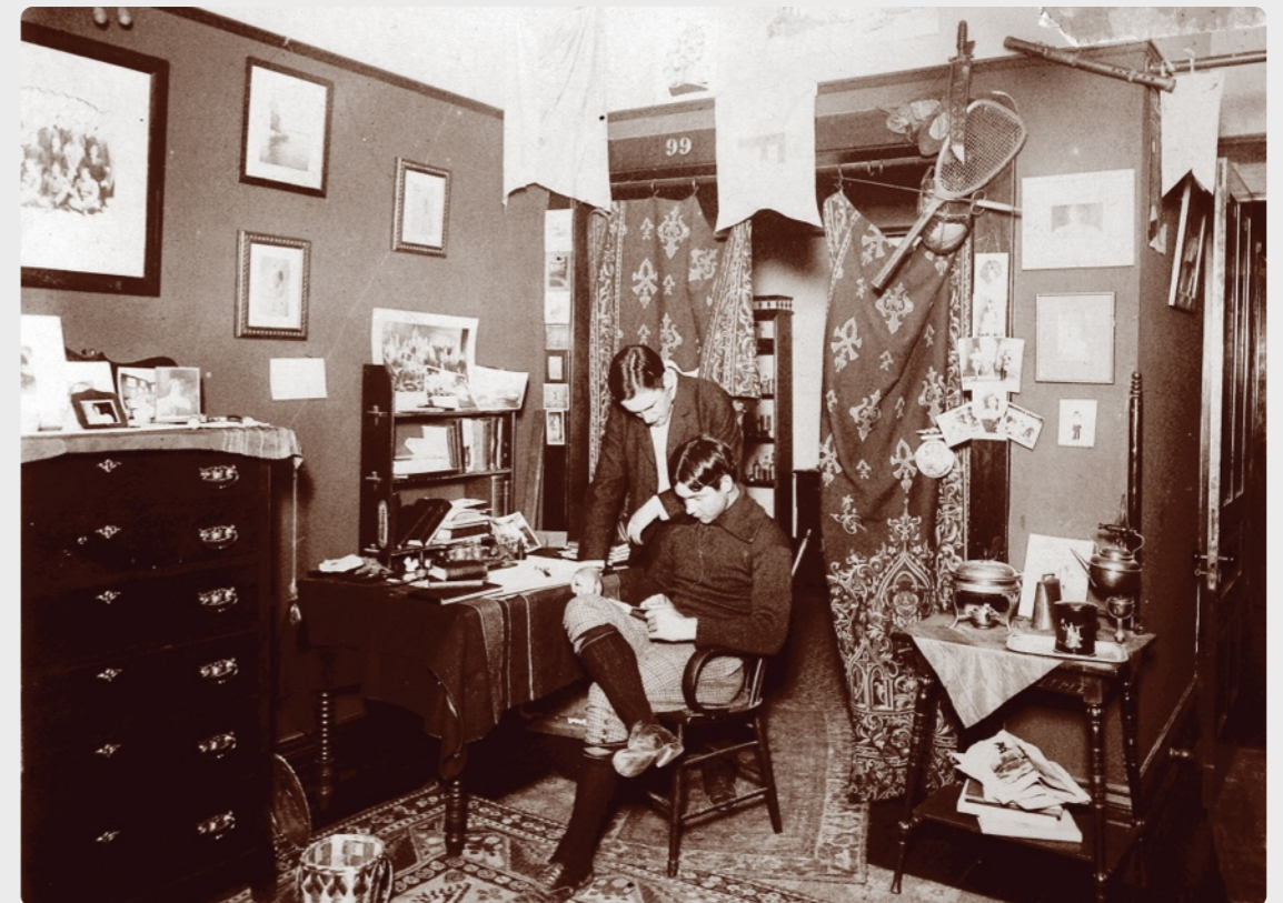
Student dormitory rooms
