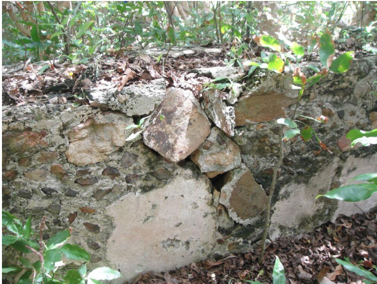
Figure 8. Closed archway of Structure F
