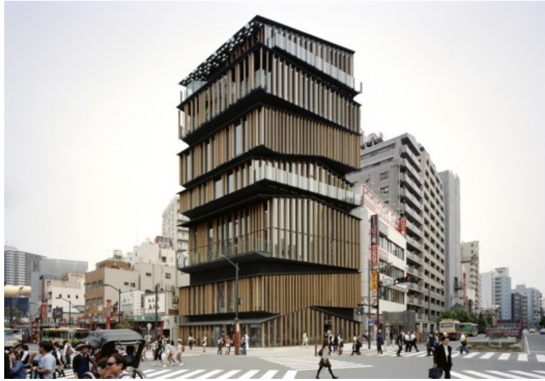
Image 88. The Asakusa Culture and Tourism Center as seen from the north side of Kaminarimon Street ( http://www.archdaily.com/251370/asakusa-culture-and-tourism-center-kengo-kuma-associates/ ).
