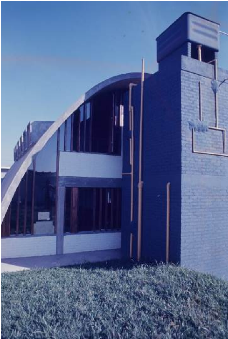
Image 26. Dino Zammataro House, Rodrigo Lefèvre, 1970. The image shows important elements of Arquitetura Nova: the arched roof, the visible structures, and the emphatic indexicality of labor in the use of mortar. Source: Unknown Photographer, 1970s, FAU-USP archives.
