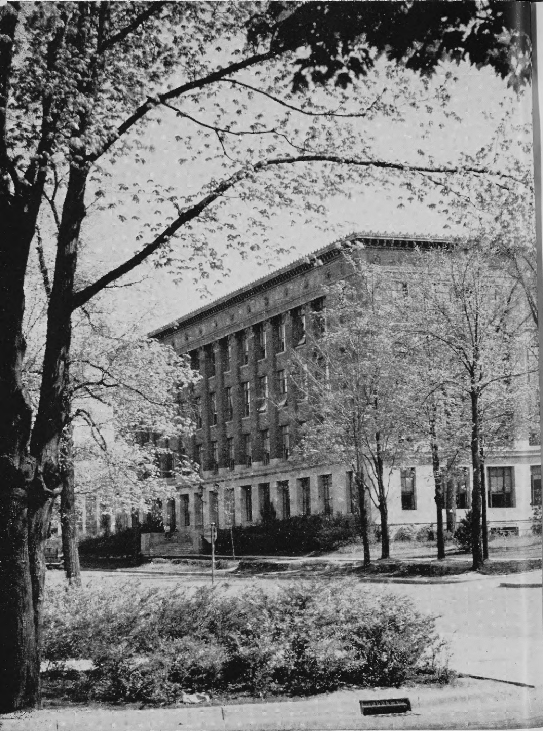
EAST ENGINEERING BUILDING
