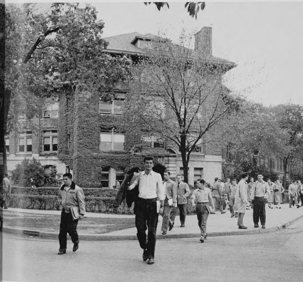
WEST ENGINEERING BUILDING
