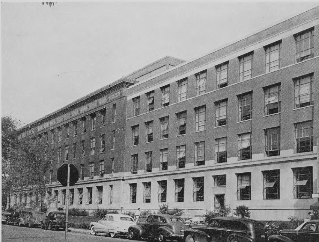
East Engineering Building
