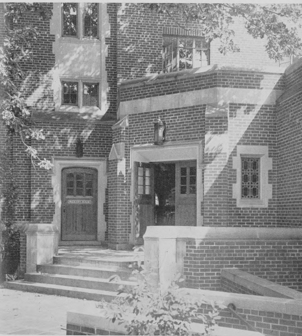
Prescott House, East Quadrangle residence for men
