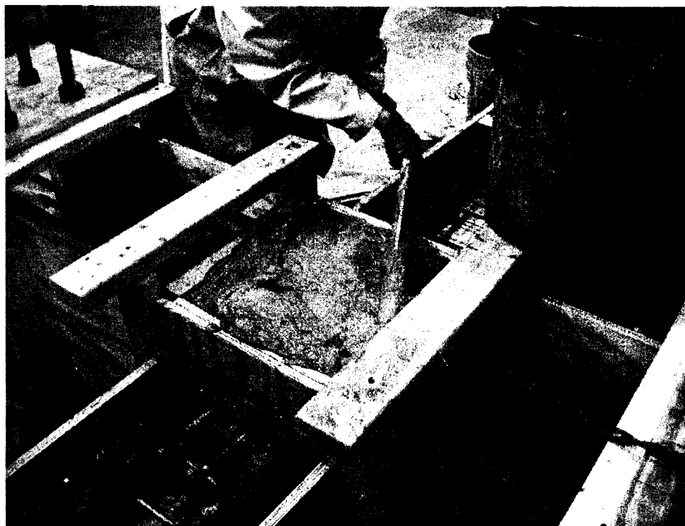
Figure 6.13 Casting and vibration of HPFRCC portion of the beam-column specimen
