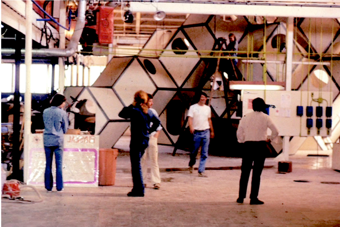
Illustration 1.13 1800 Berkeley Street, renovations, c. 1972 (image courtesy of SCI-Arc).
