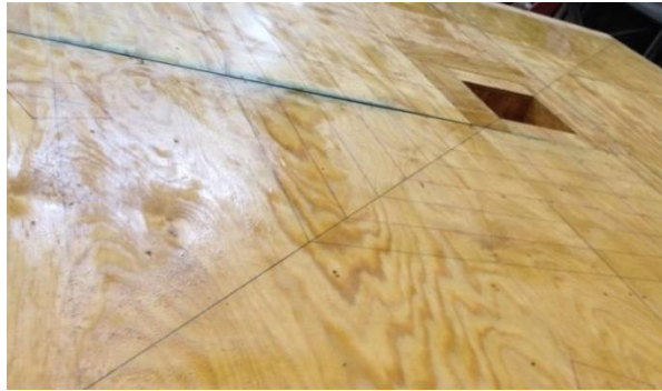
a. Oil treatment for formwork
