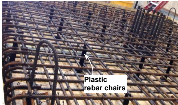
c. Top slab reinforcement installation
