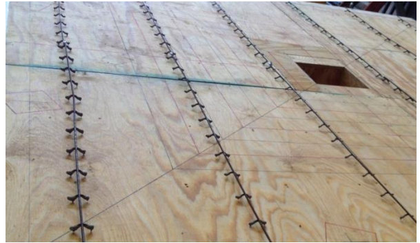
b. Slab bolsters placement
