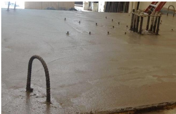
c. Surface leveling
