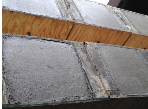
Fig. 3-10: Cast concrete for supporting blocks.
