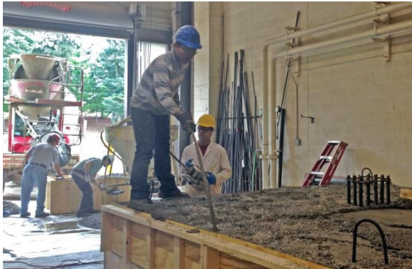
a. Pouring and vibrating
