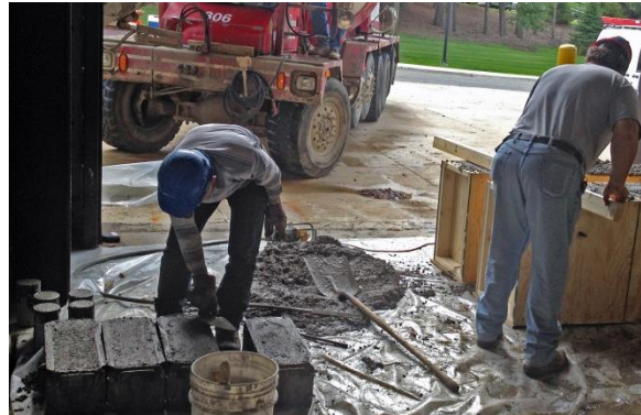
b. Concrete cylinders and beams making
