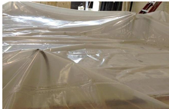
d. Concrete curing
