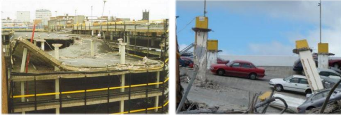
Fig. 1-4: Collapse of flat plate buildings due to punching shear failure
