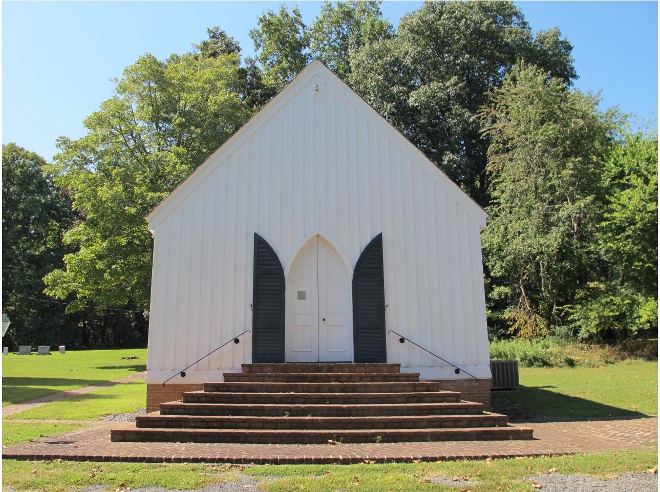
Figure 2.2: Chapel from Bremono Plantation, Fluvanna County, Virginia
