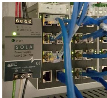
Figure 24: UPS Ethernet connectivity: Modbus IP
