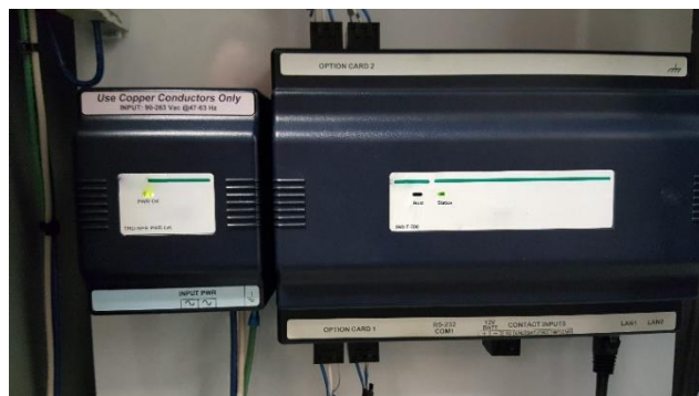
Figure 28: Aggregate controllers
