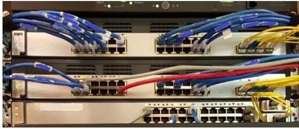
Figure 29: Switch stack
