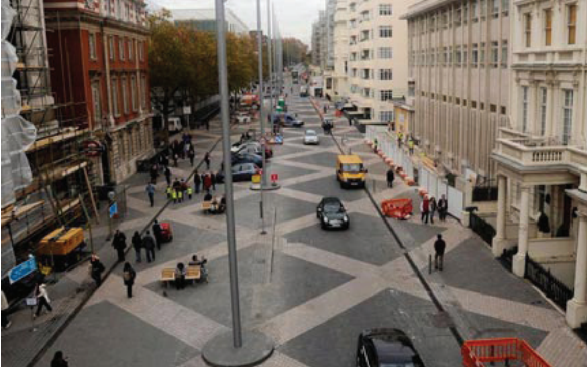
Figure 3-4: Lightpoles and trench drains provide structure and coherence on Exhibition Road. Source: London Living.
