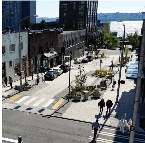
Figure 6-3: Bell Street Park in Seattle is a shared street that aims to infuse public space in a densely built area of the city. Source: SvR Design
