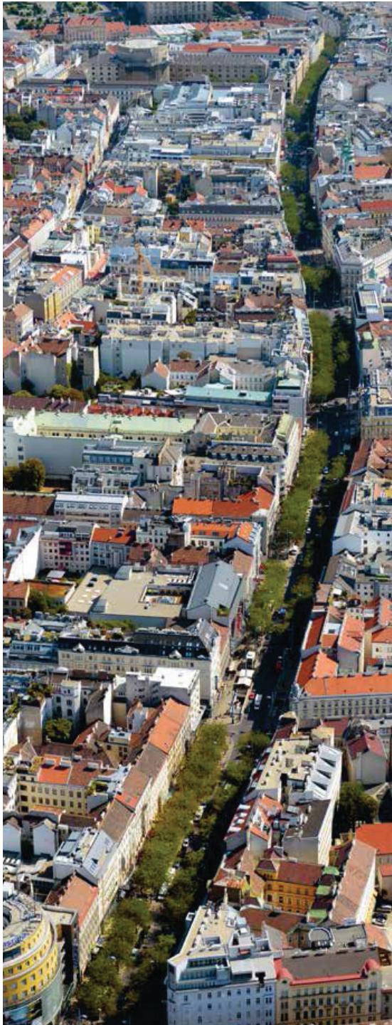
Figure 5-1: Aerial photo of the Mariahilferstrasse looking east toward the Museum Quarter. Source: Christian Fürthner
