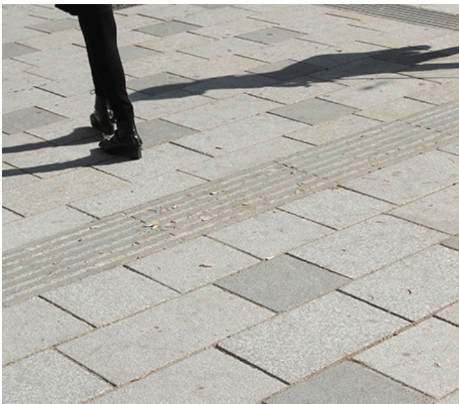
Figure 5-13: Textured tactile pavement communicates safe zones to the visually impaired. Source: FCP
