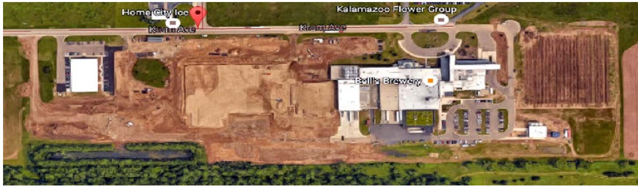
Figure 5.9.1: Aerial Image of Comstock Facility
