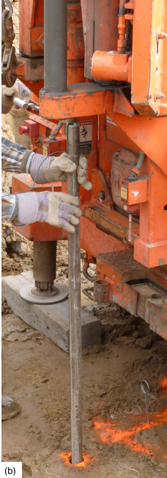
Figure 5-15 (a) Feeding of cable through the rod and (b) attachment of drill rig with rod
