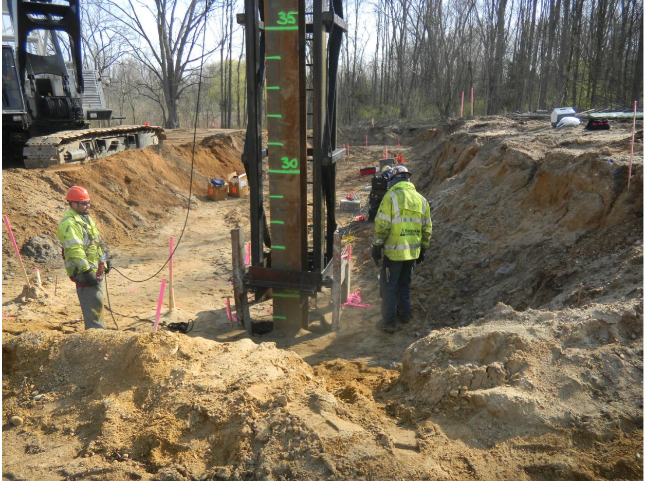
Figure 6-14 Pile driving at US-131 site at bridge abutment A
