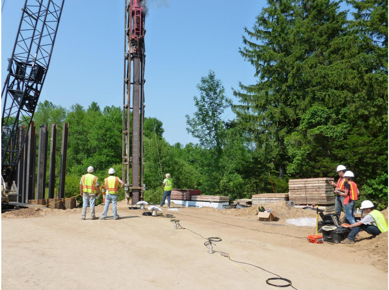
Figure 6-8 Pile driving at M-25 site
