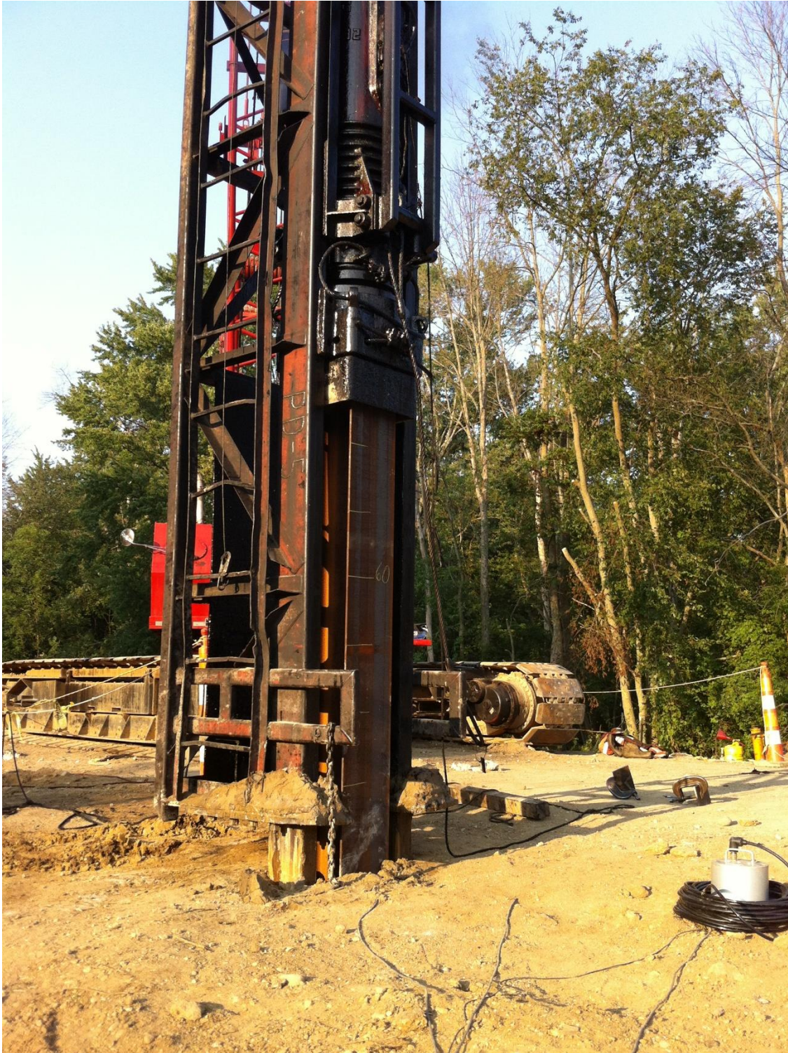
Figure 6-11 Pile driving at M-66 site
