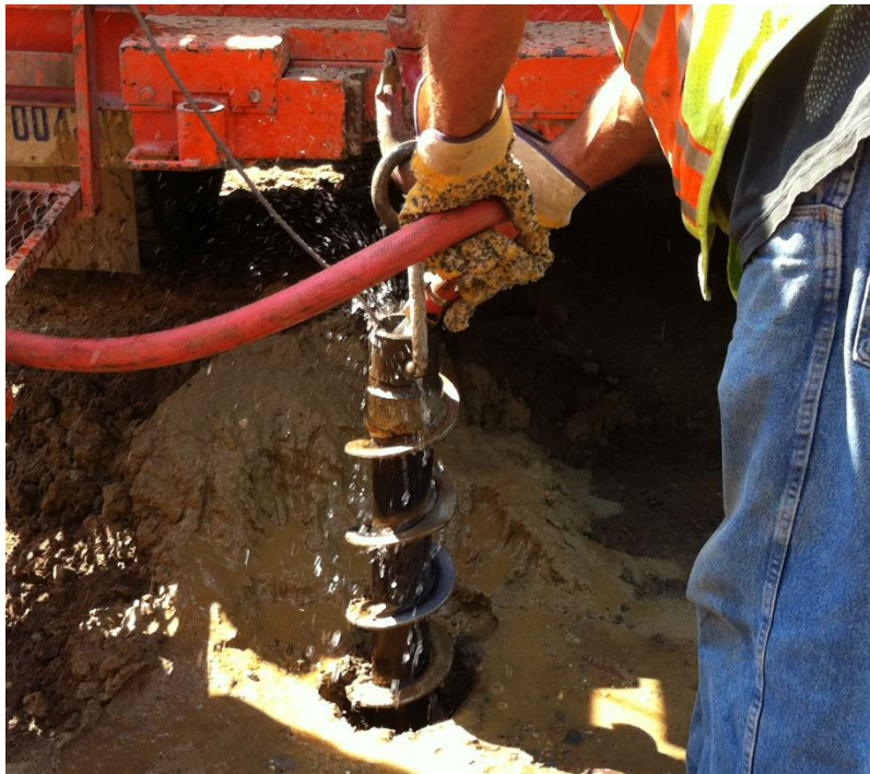
Figure 5-13 Withdrawal of the hollow stem flight auger
