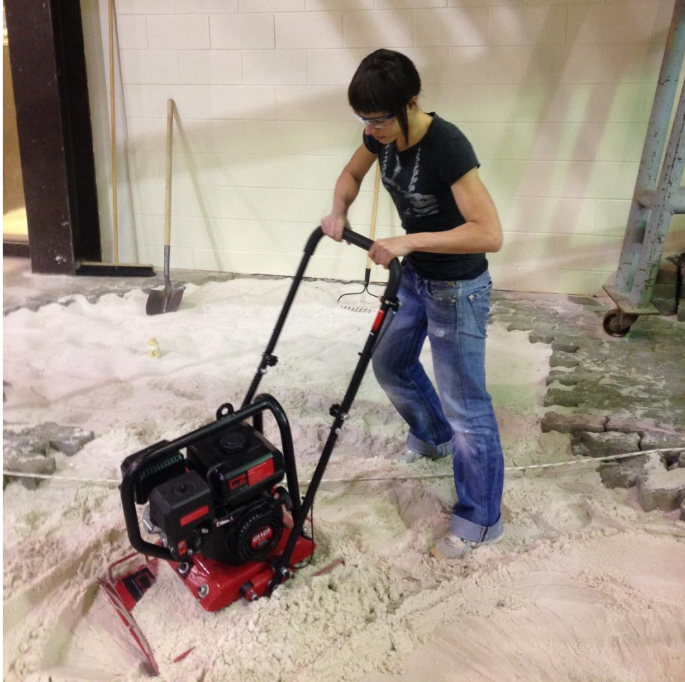
Figure 8-10 Compaction of silica sand using a vibratory plate compactor
