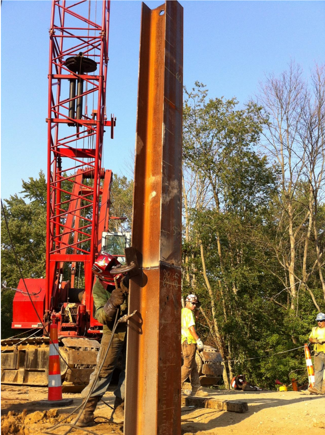
Figure 6-10 Welding a pile section on the test pile of M-66 site
