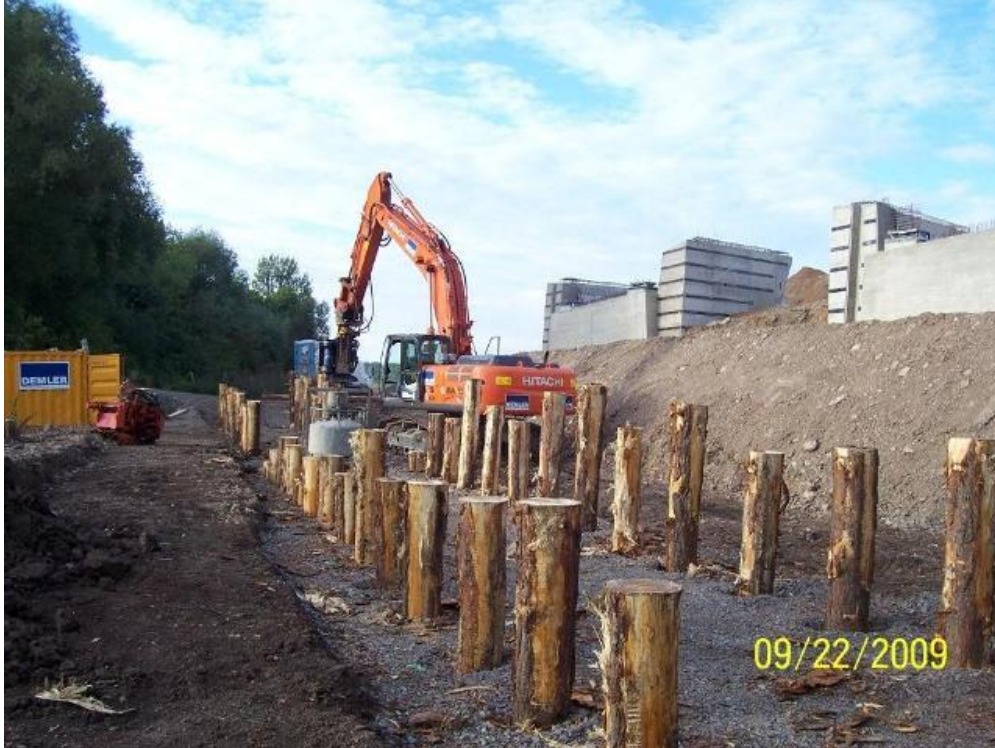
Figure 4-1 Installation of timber piles (Courtesy of DEMLER Spezialtiefbau GmbH and Co.)
