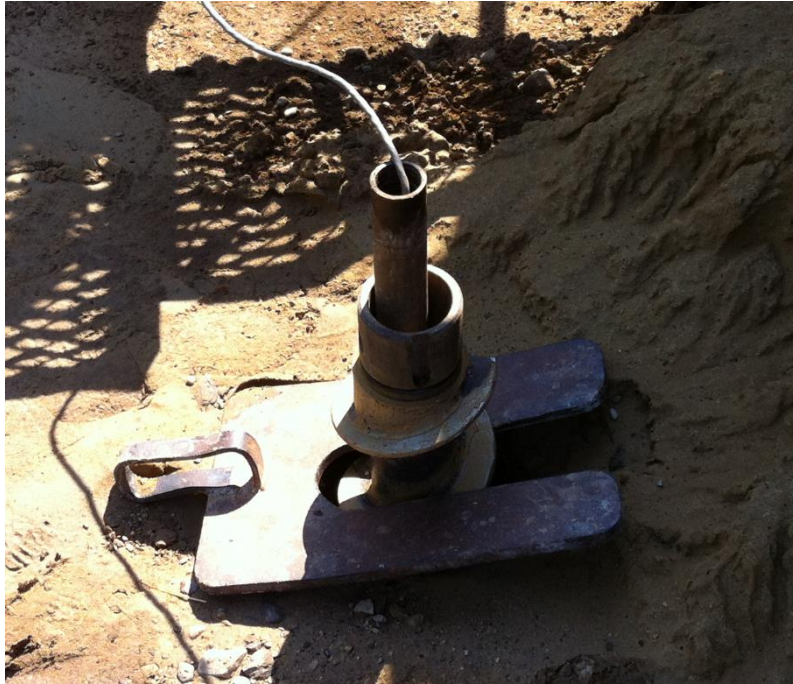
Figure 5-12 SPT rod inside the hollow stem flight auger
