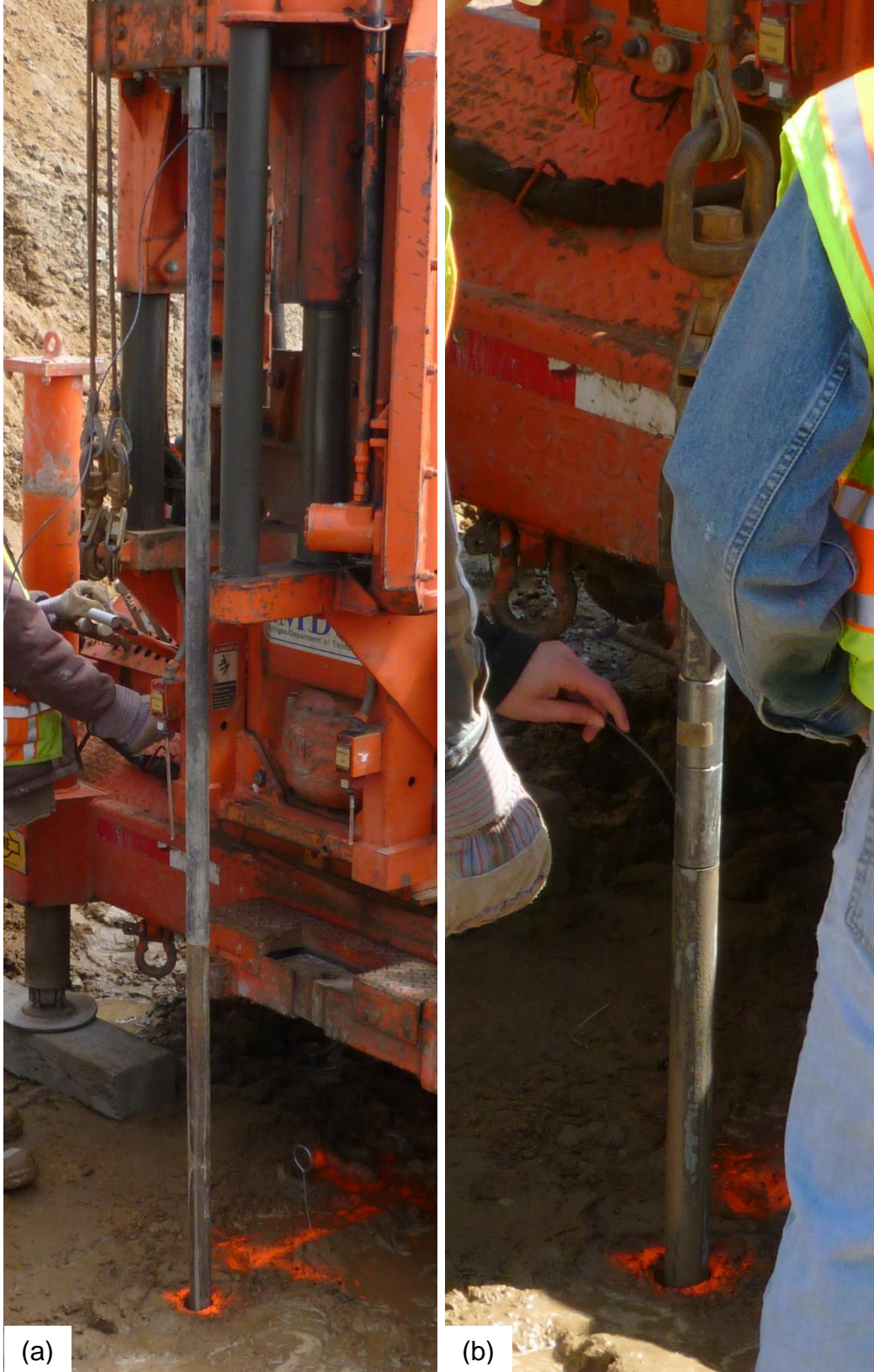
Figure 5-16 (a) Pushing the rods and (b) rod extraction
