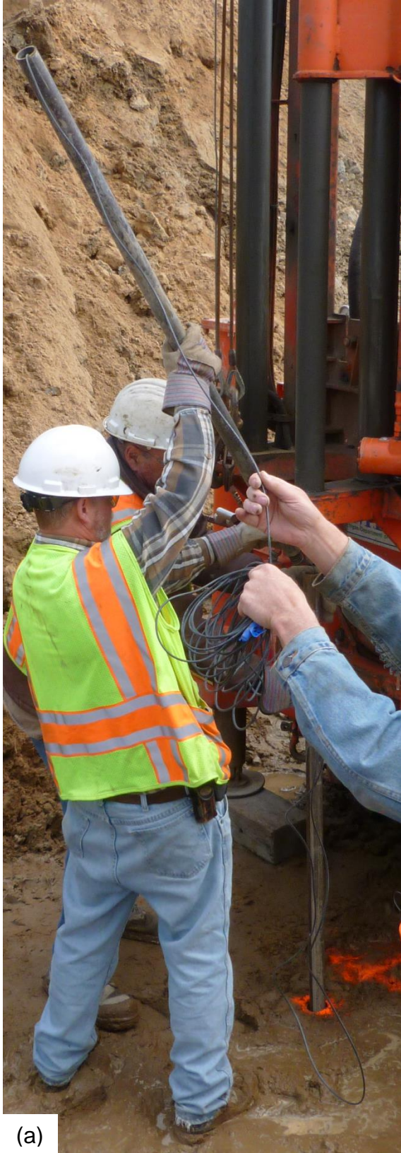
Figure 5-15 (a) Feeding of cable through the rod and (b) attachment of drill rig with rod
