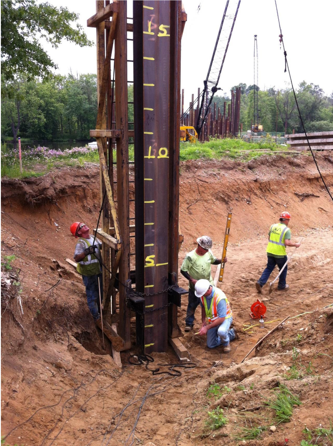
Figure 6-17 Positioning of pile #54 at US-131 site at bridge abutment B
