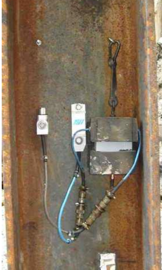
Figure 4-22 Accelerometer (left), strain gage (middle) and transmitter mounted near the top of an H-pile (Pile Dynamics, Inc.)
