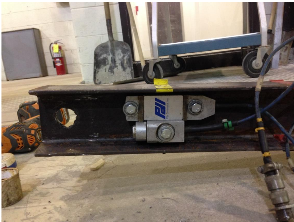
Figure 8-20 Accelerometer and strain gage mounted near the top of the pile
