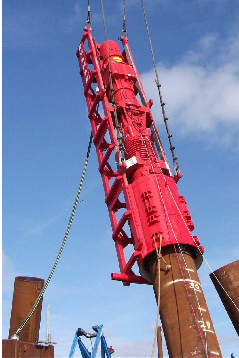
Figure 4-16 Diesel hammer driving pipe steel piles (courtesy of Delmag)
