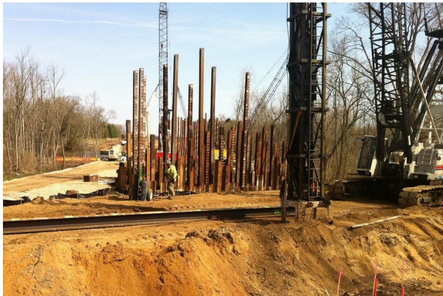
Figure 4-6 H-piles in one of the tested sites for this project
