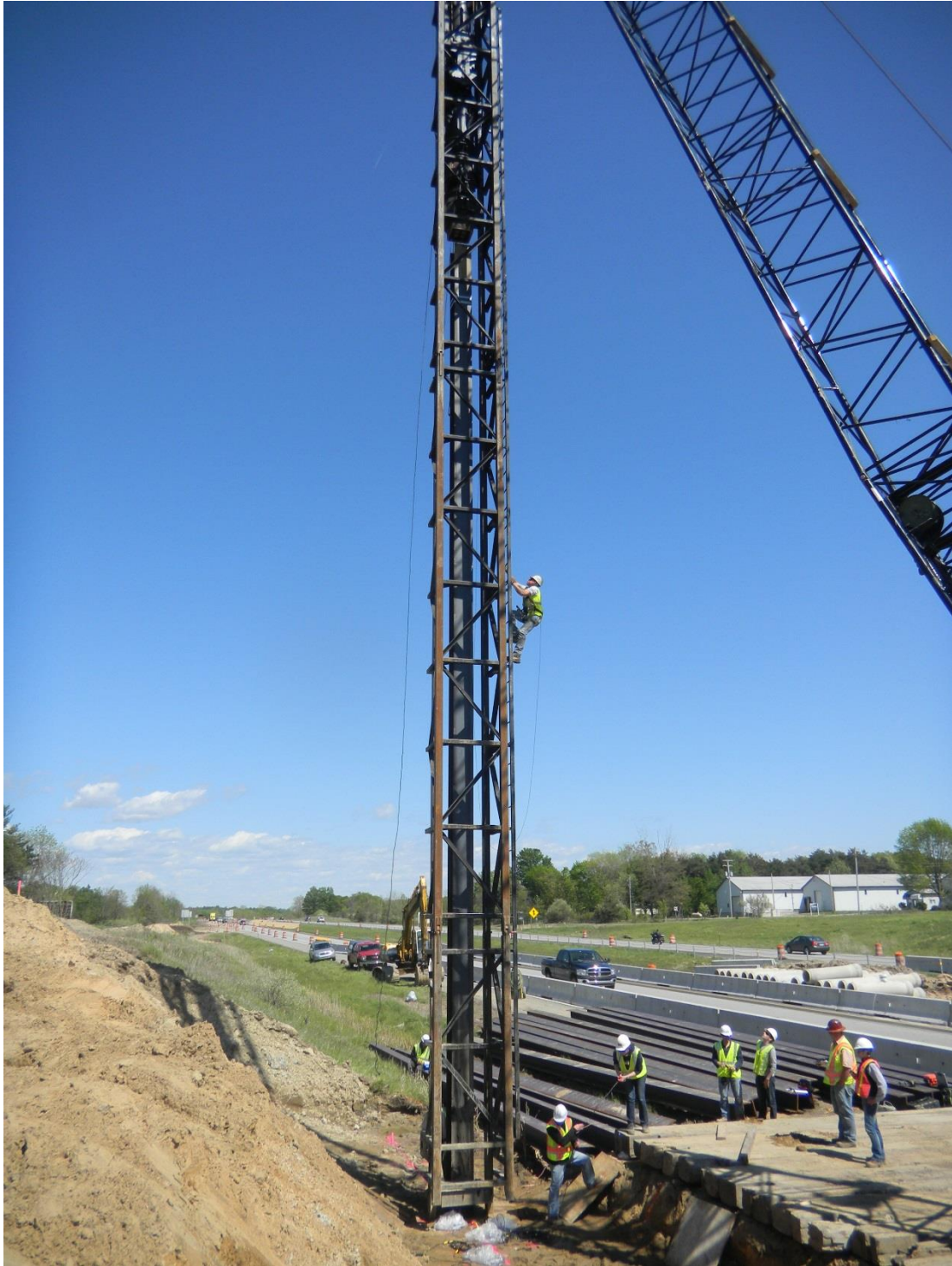
Figure 6-7 Spotting the pile at I-96 site
