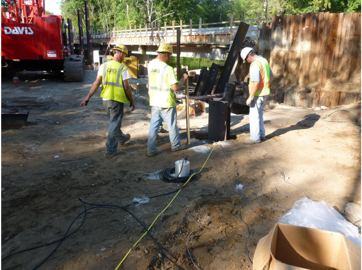
Figure 6-12 Test pile after the end of driving at M-139 site
