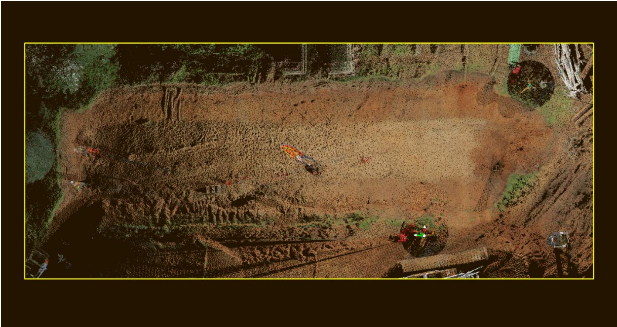
G 4 TOP SCREEN CAPTURE AT ABUTMENT B OF US-131 SITE
