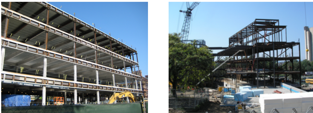
Figure 2.1 Examples of Steel Moment Frame Construction ( www.ecs.umass.edu )
