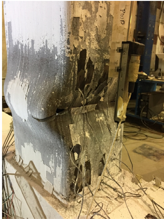
Figure 4.20 Fracture Propagation at Beam Corners of Collar Connection without Stiffeners at the End of the 0.08 rad. Rotation Cycle
