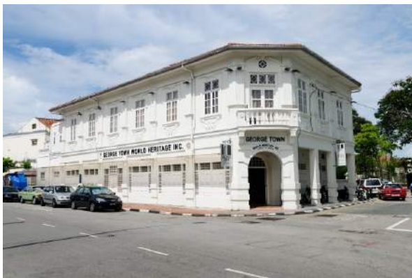
Figure 4.24a: GTWHI office building (source: GTWHI)
