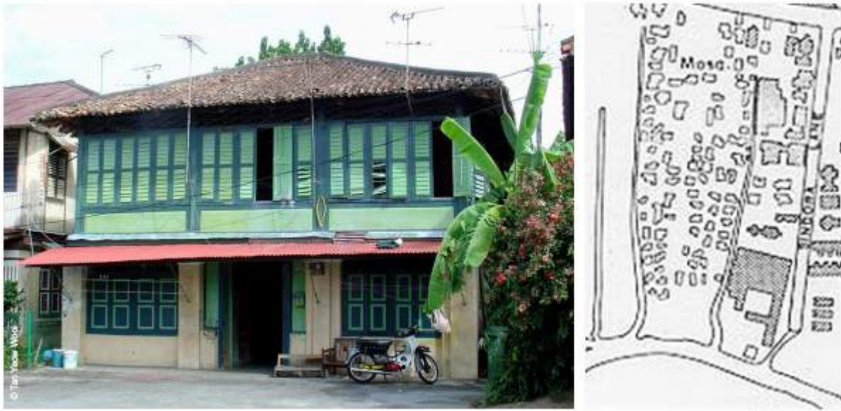
Figure 4.6: George Town bungalow, a standalone building type (source: SAP)
