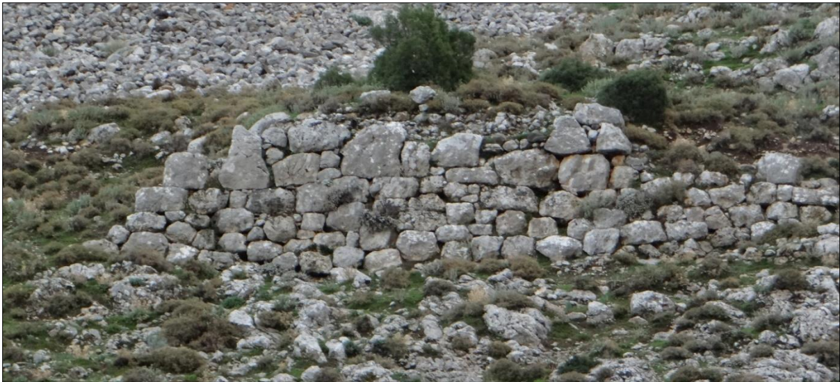
Figure 51: View of fortification wall at Palaiopyli on Kos, probably of LH III date (Photo author).
