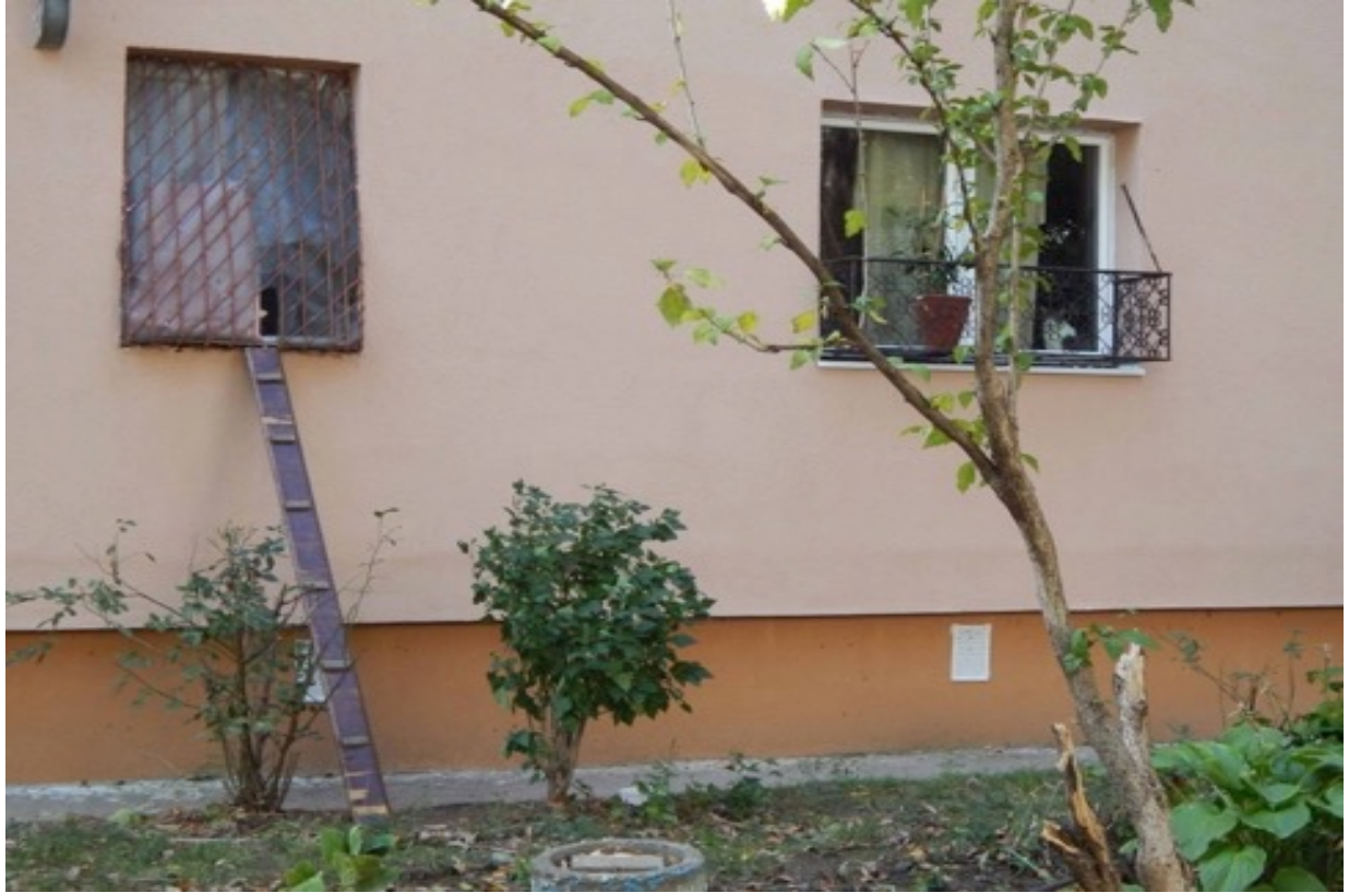
Figure 44: Ladder to the kitchen.
