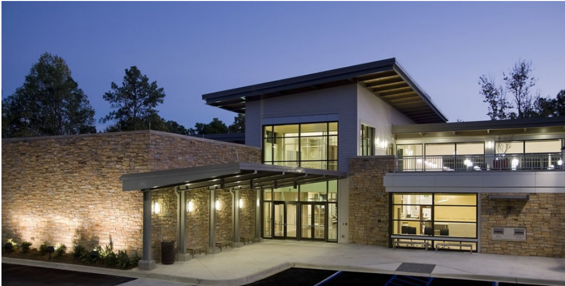
Figure 6.1: Front view of VHPL showing main floor entry and upper floor access to rooftop terrace. Photo courtesy of Charles Beck.
