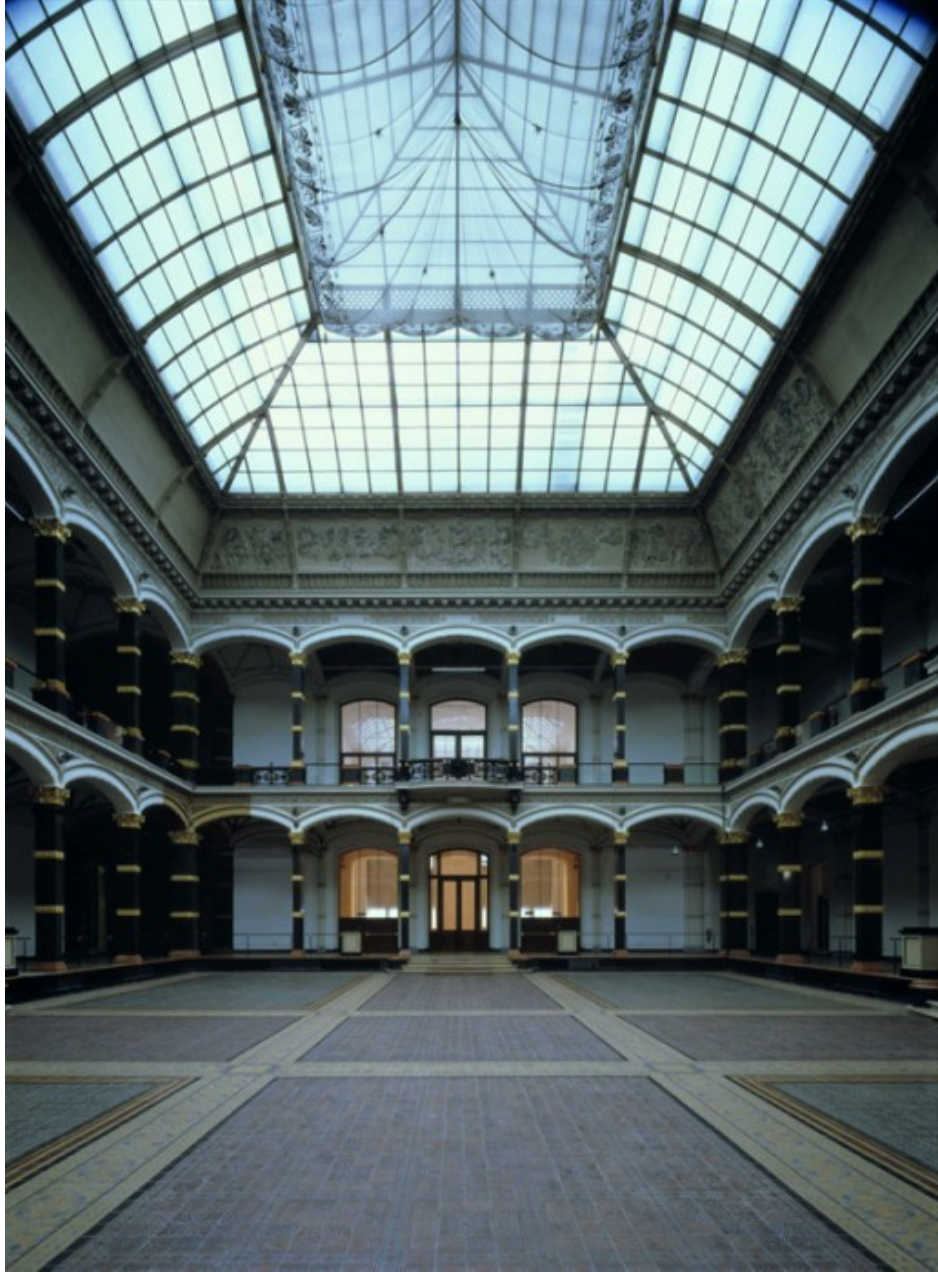
Figure IV.2: Atrium at the Martin-Gropius-Bau, formerly the Kunstgewerbemuseum, Berlin.
