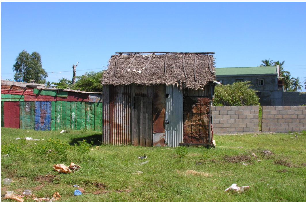
Figure 49: Home constructed of sheet metal (toly), steel drums (barika), with thatch and wood roof, Andovinjo, Mahajanga, 2014, (Source: Author)
