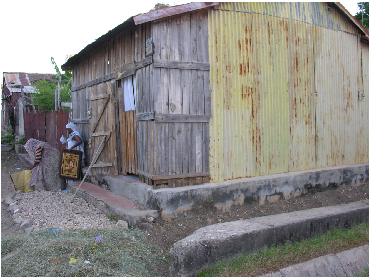
Figure 50: Trano toly (sheet metal home), with concrete floor, and wooden baraza on front side, Morafeno (Source: Author)
