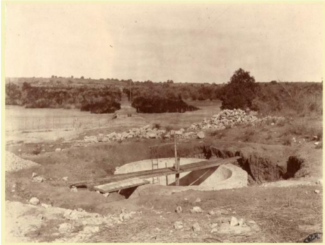
Figure 71: Construction of a well, Majunga 1903 (Source: Archives Nationales d'outre mer, Fonds Gallieni, FR ANOM 44PA 134/8)
