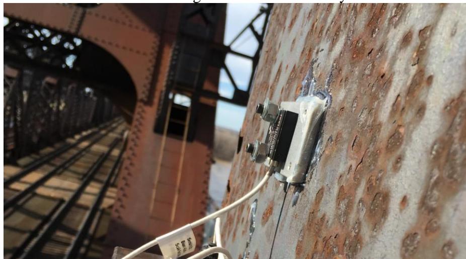
Figure 3.14 Uni-axial accelerometers installed on eyebar portion of MS0 – US0.
