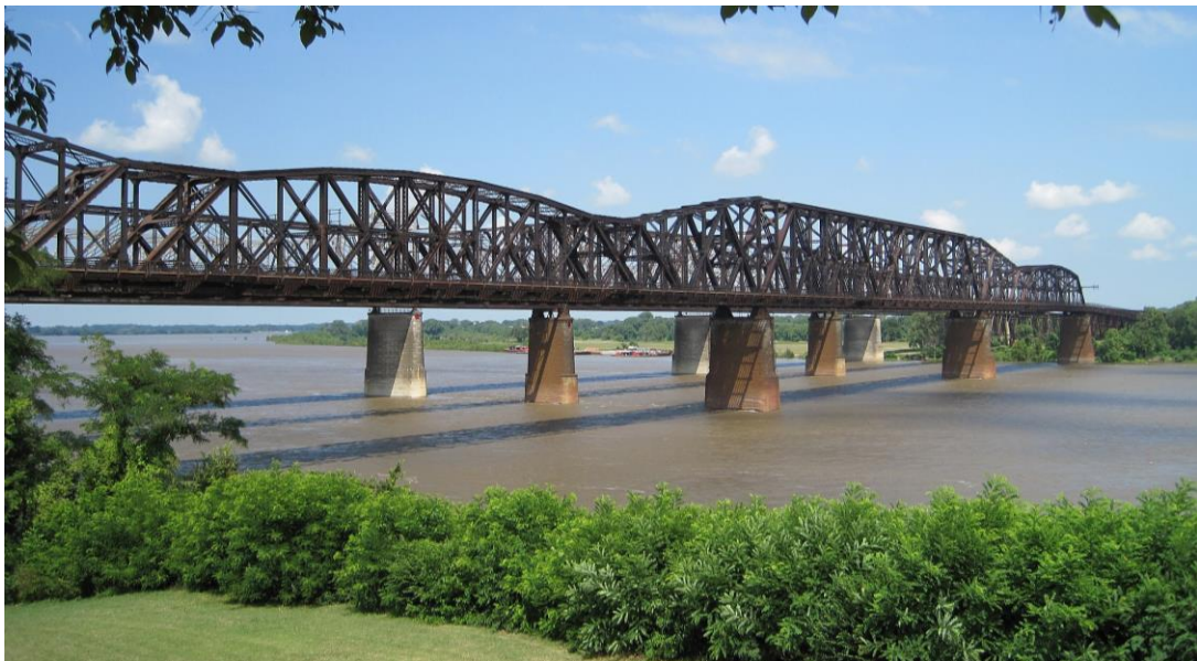
Figure 3.3 View of Harahan Bridge looking south from east bank (Machnitzki 2010).
