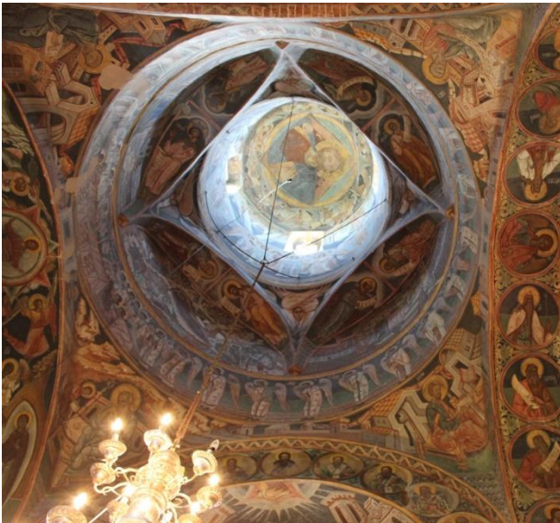
Figure 3.11 Detail of tower, interior, Church of St. Nicholas, Probota Monastery (source: author)
