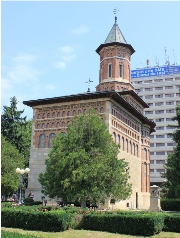
Figure 3.59 Church of St. Nicholas, Iași, Moldavia, 1491-1493, view from SW (source: author)
