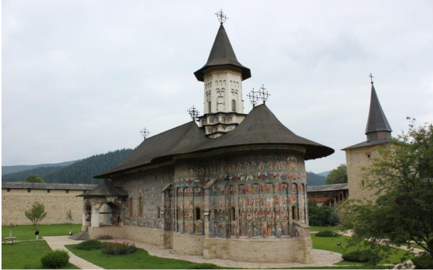
Figure 7.1 Church of the Resurrection, Sucevița Monastery, Moldavia, 1581-1583, view from SE (source: author)
