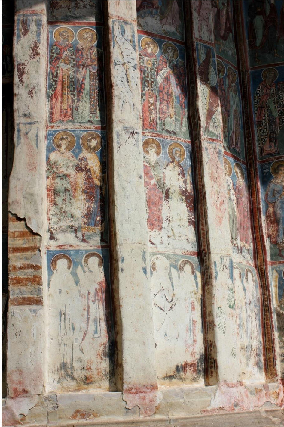
Figure 4.11 Brick and stone underpainting, south wall, Church of the Dormition of the Virgin, Humor Monastery (source: author)
