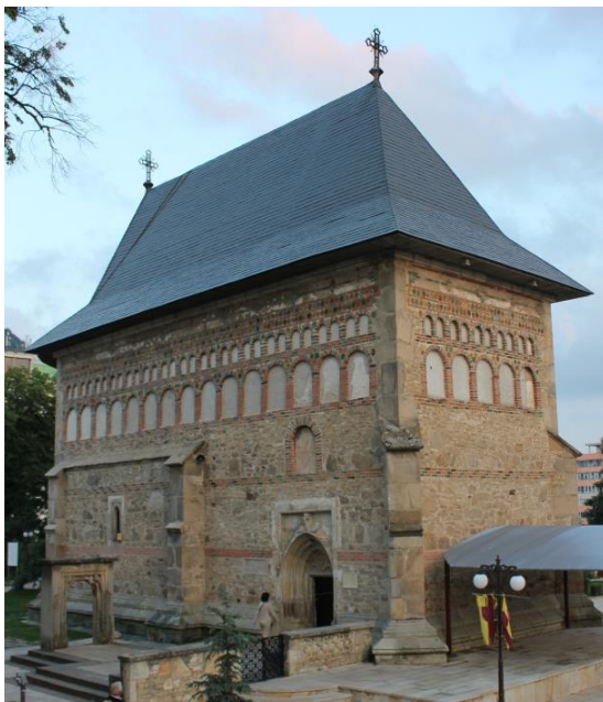
Figure 3.96 Exterior buttresses, north wall, Church of St. John the Baptist, Piatra Neamț (source: author)
