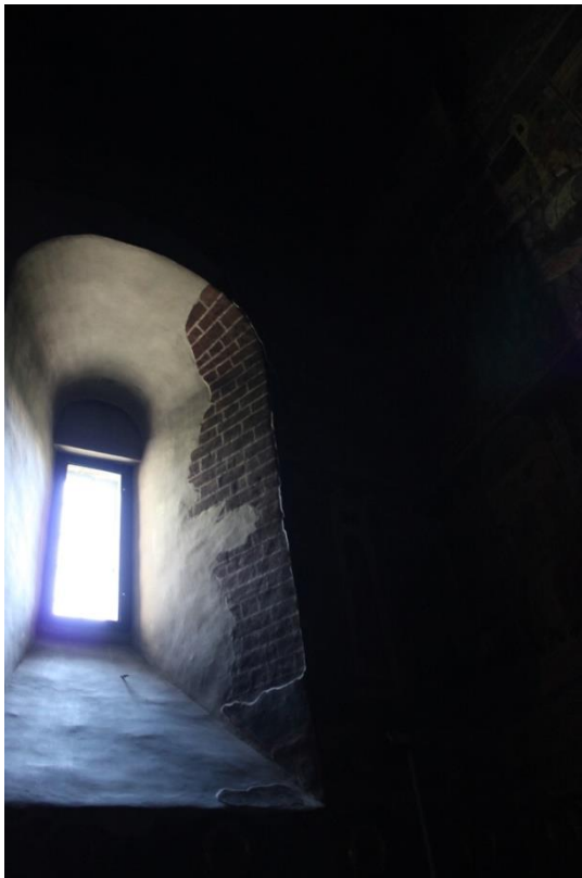
Figure 4.4 Brick underpainting, south window, burial chamber, Church of the Ascension, Neamț Monastery (source: author)
