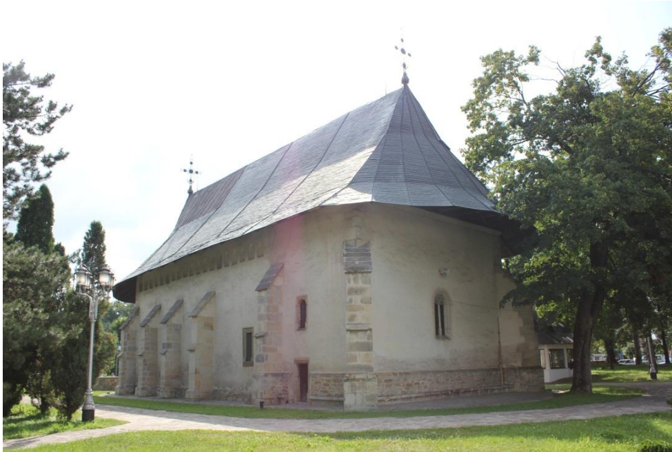
Figure 3.122 Church of St. Nicholas, Rădăuți Monastery, Moldavia, 1367-1368, view from NW (source: author)
