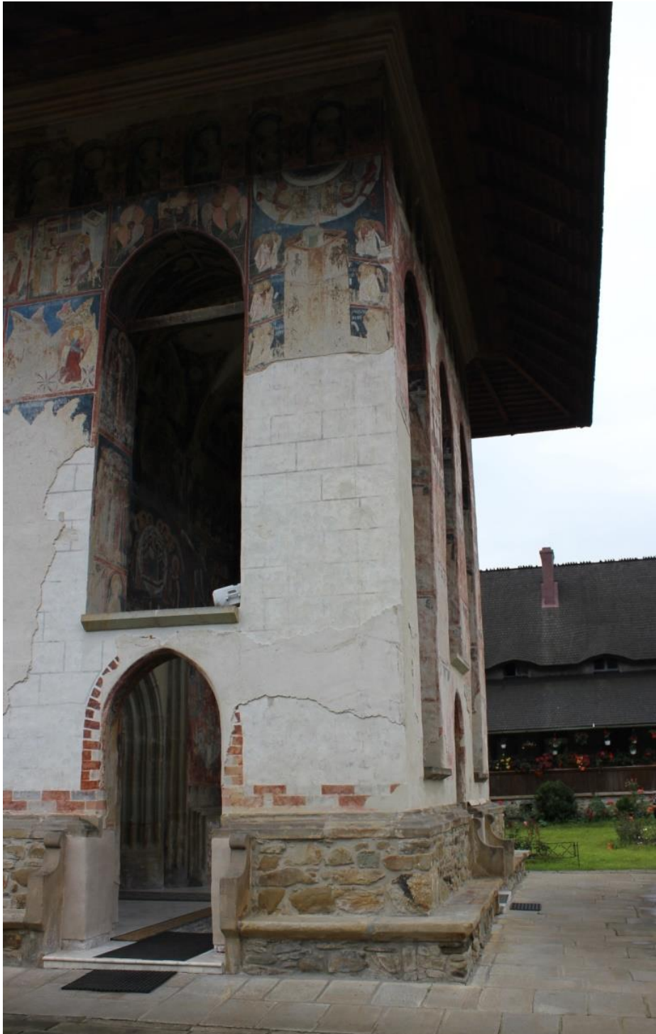
Figure 4.6 North wall, Church of the Annunciation, Moldovița Monastery (source: author)
