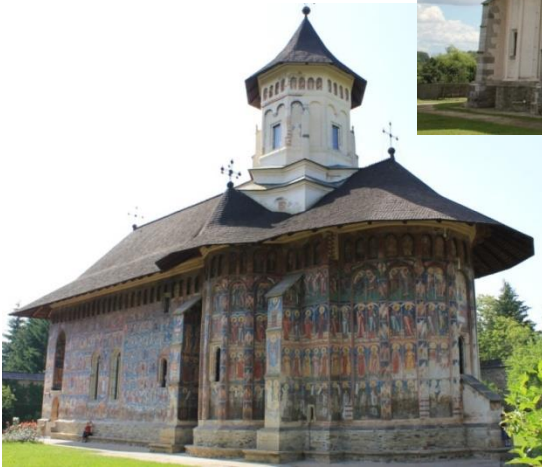
Figure 3.98 Exterior buttresses (source: author)
