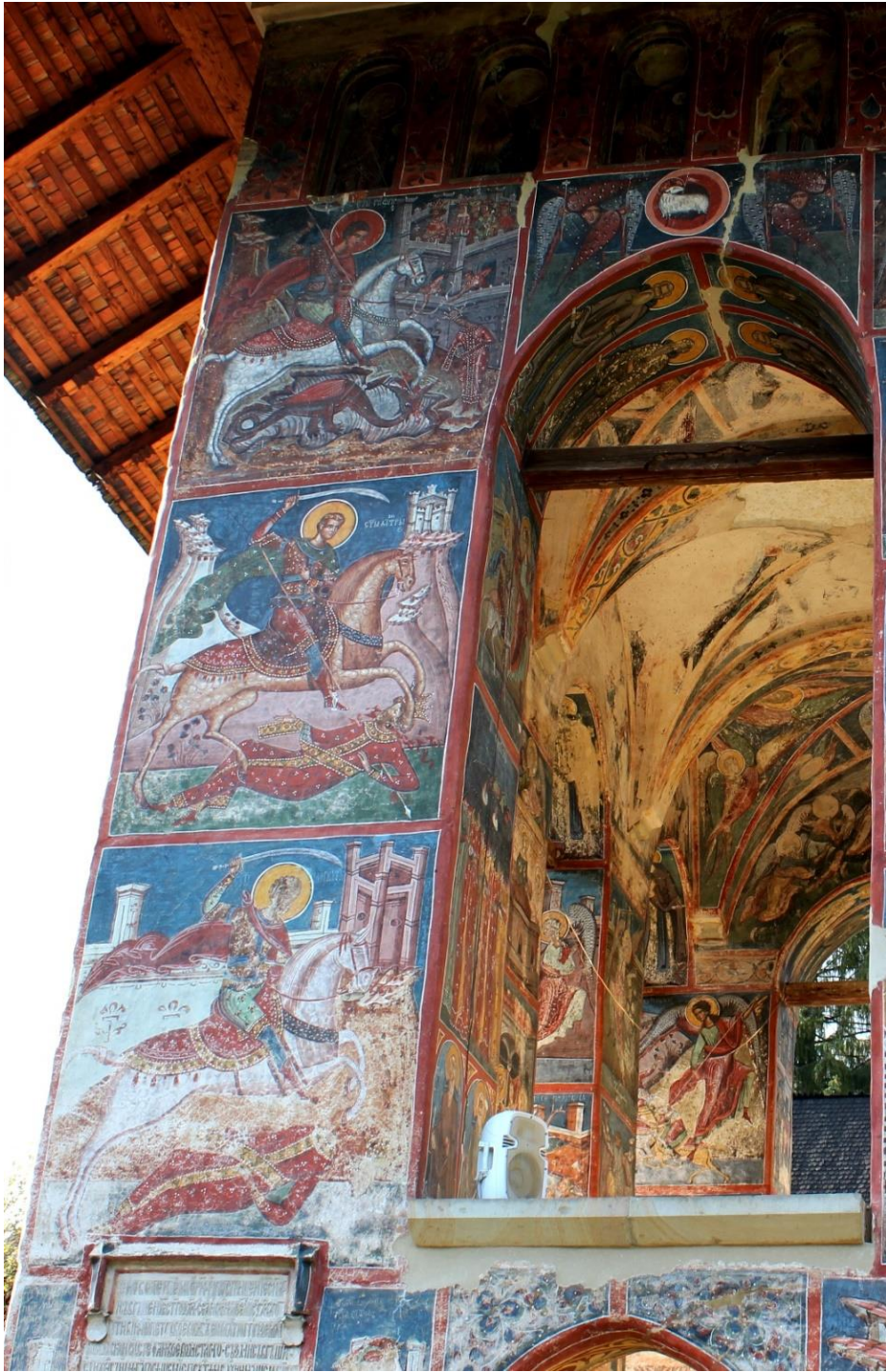
Figure 4.85 West pillar, south wall, Church of the Annunciation, Moldovița Monastery (source: author)
