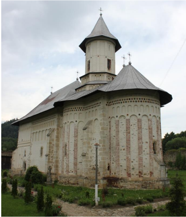
Figure 3.95 Exterior buttresses, south wall, Church of the Birth of the Virgin, Tazlău Monastery (source: author)
