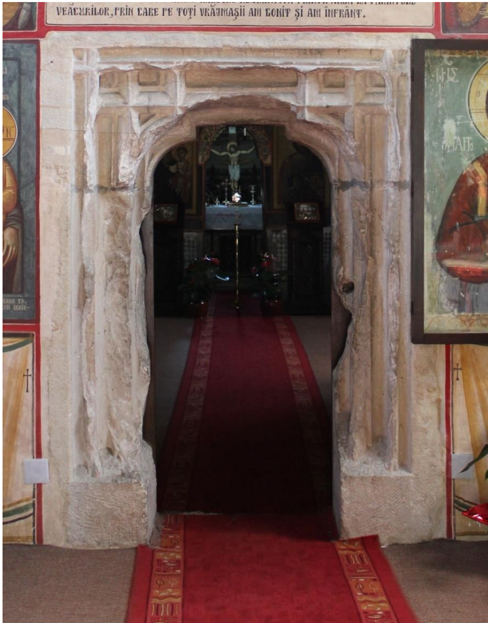
Figure 3.107 Schulterbogenportal, interior, threshold between pronaos and naos, Church of the Dormition of the Virgin, Borzești (source: author)
