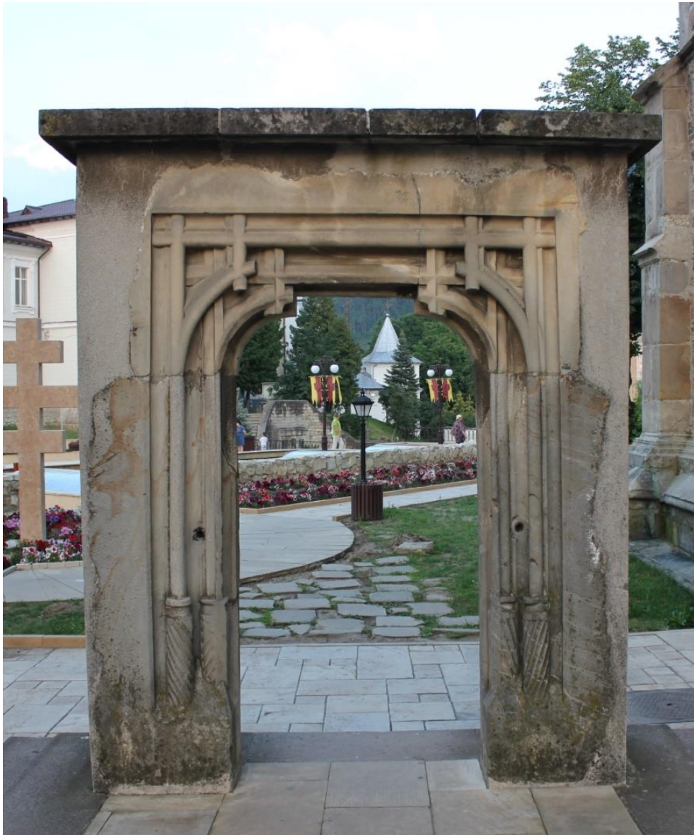
Figure 3.106 Schulterbogenportal, originally in the interior at the threshold between pronaos and naos, now outside of the church, Church of St. John the Baptist, Piatra Neamț (source: author)
