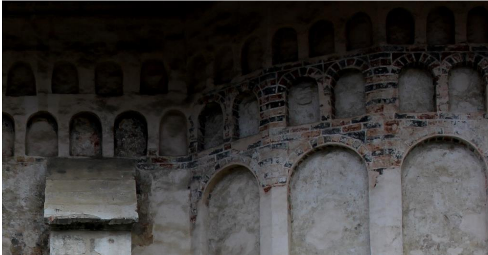
Figure 4.3 Painted brick exterior, south wall, Church of St., Demetrios Suceava (source: author)
