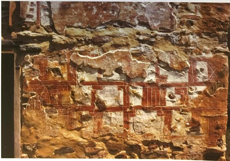
412 Kurbinovo, St. George; west façade; detail of painted building opus
