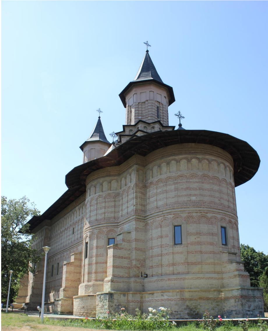
Figure 3.97 Exterior buttresses, south wall, Church of the Ascension, Galata Monastery (source: author)
