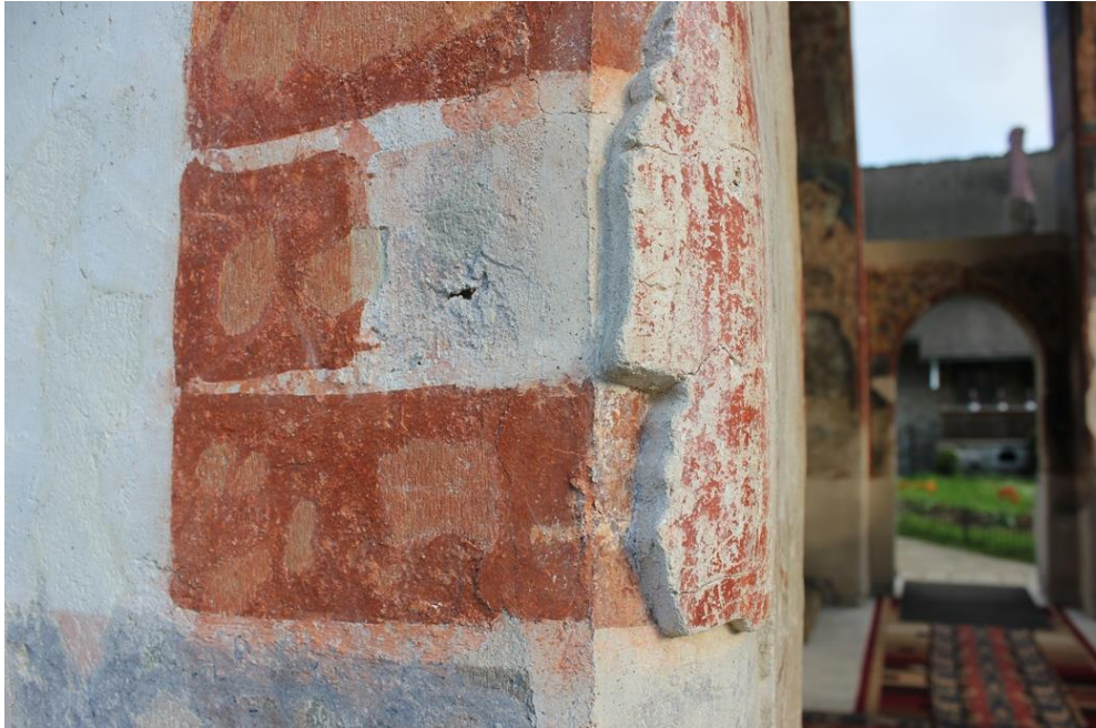
Figure 4.7 North wall, Church of the Annunciation, Moldovița Monastery (source: author)
