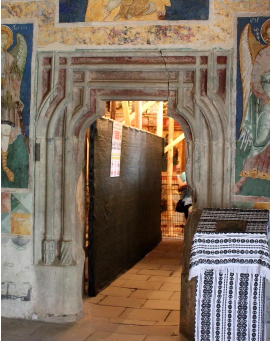
Figure 3.108 Schulterbogenportal, interior, threshold between pronaos and naos, Church of the Beheading of St. John the Baptist, Arbore (source: author)
