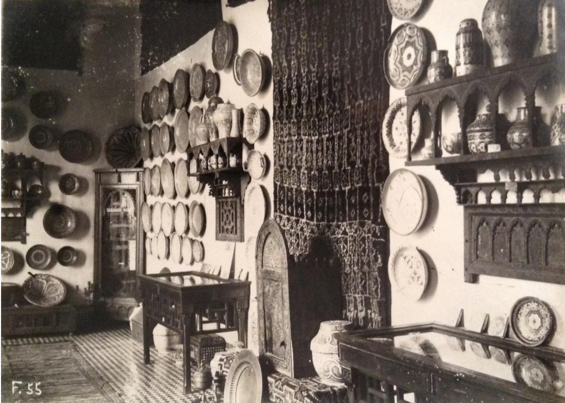
Figure 2.4: The faience room in Dar Batha Museum, Fez (ca. 1920). Photograph mounted to an album page, Archives DPC-Maroc.
