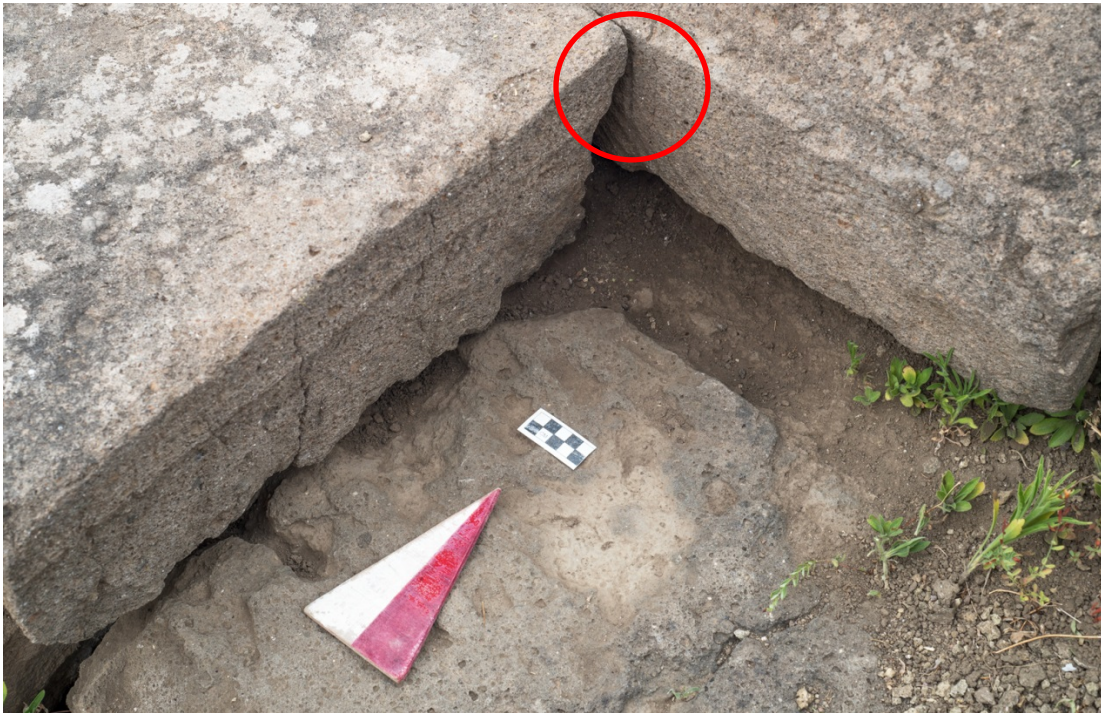
Figure 22: Vertical setting line on block of staircase in front of Temple A, 5 cm scale (author).
