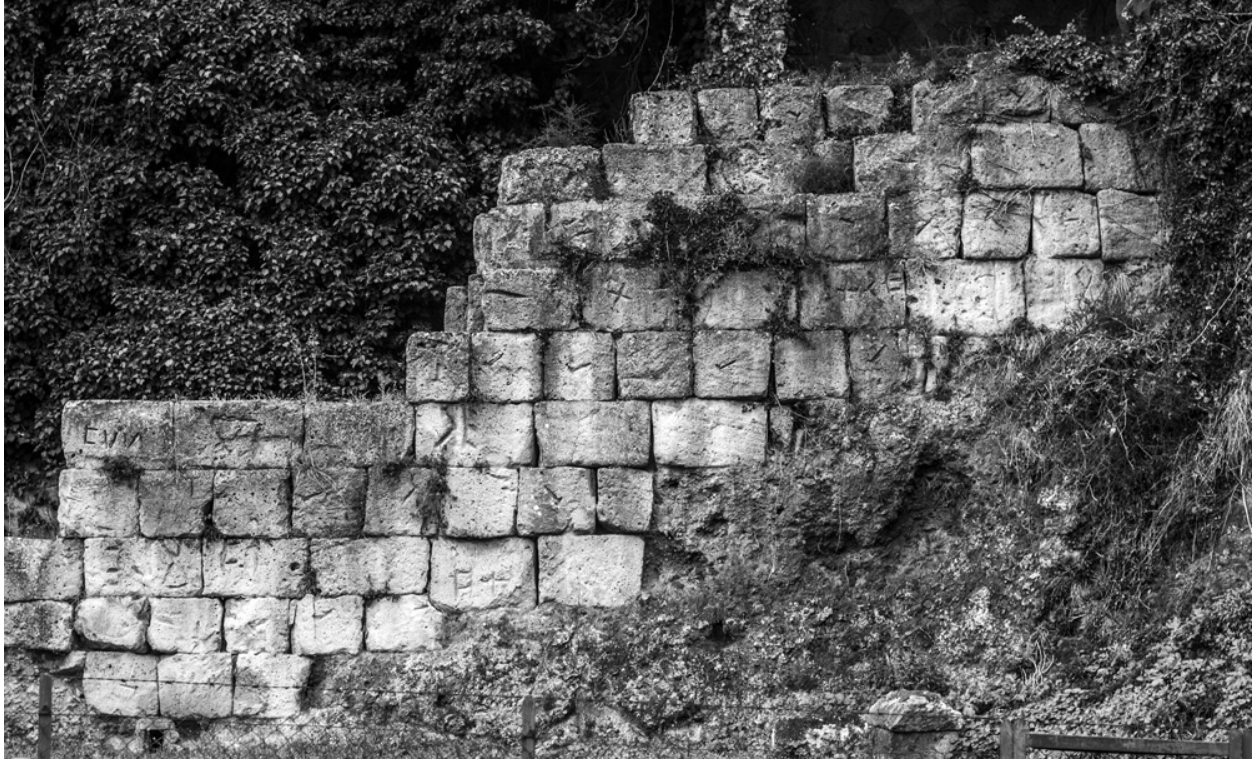
Figure 15: Quarry marks on blocks of the circuit wall at Bolsena/Volsinii Novi (author).
