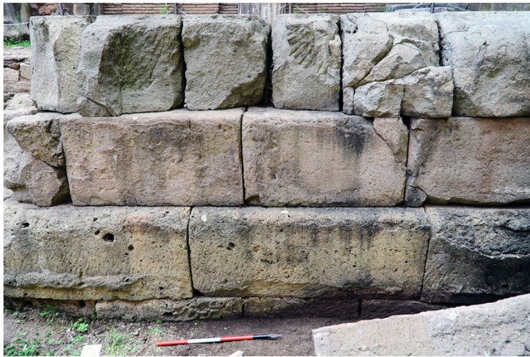
Figure 12: Sant'Omobono, east face of podium, combination of (from bottom to top) two courses of Tufo Giallo, one course each of Tufo Lionato (Anio facies) and Lapis Albanus (author).
