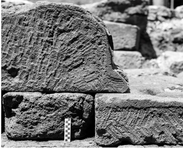
Figure 23: Anathyrosis on Lapis Albanus blocks of the eastern altar, 10 cm scale (author).
