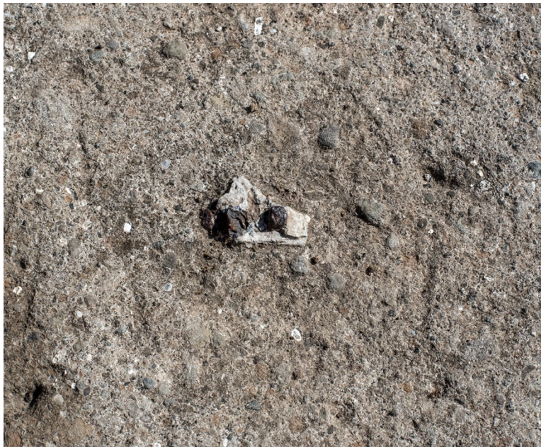
Figure 40: Close-up of fitting in Figure 39 (author).
