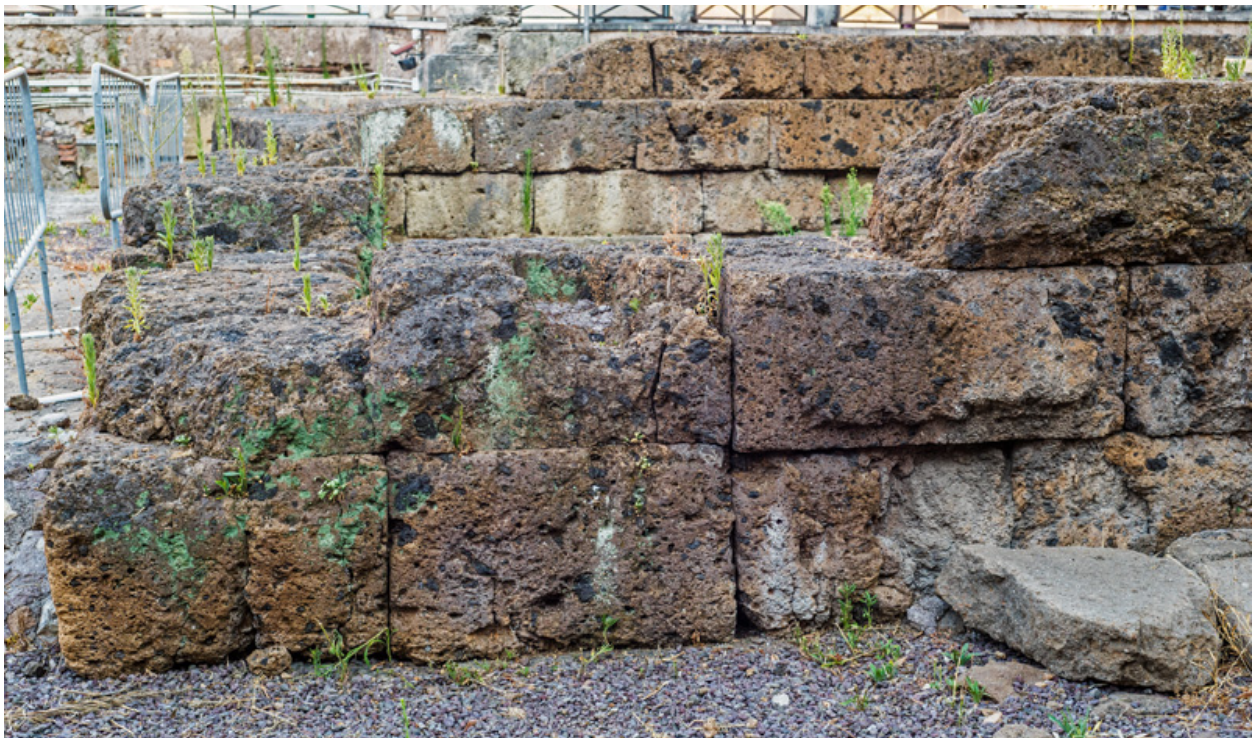
Figure 78: Southeastern corner of western cella, looking west, showing sabre cut and, to the left of it, probable replaced blocks, 2016 (author).
