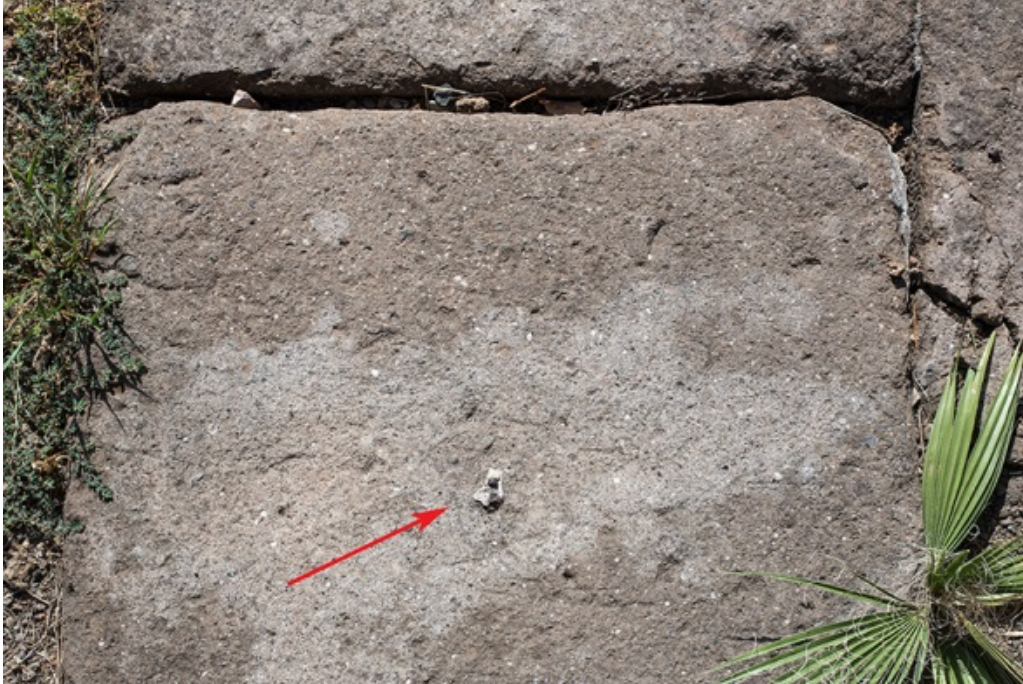
Figure 39: Lead-lined iron fitting in Anio pavement slab (author).
