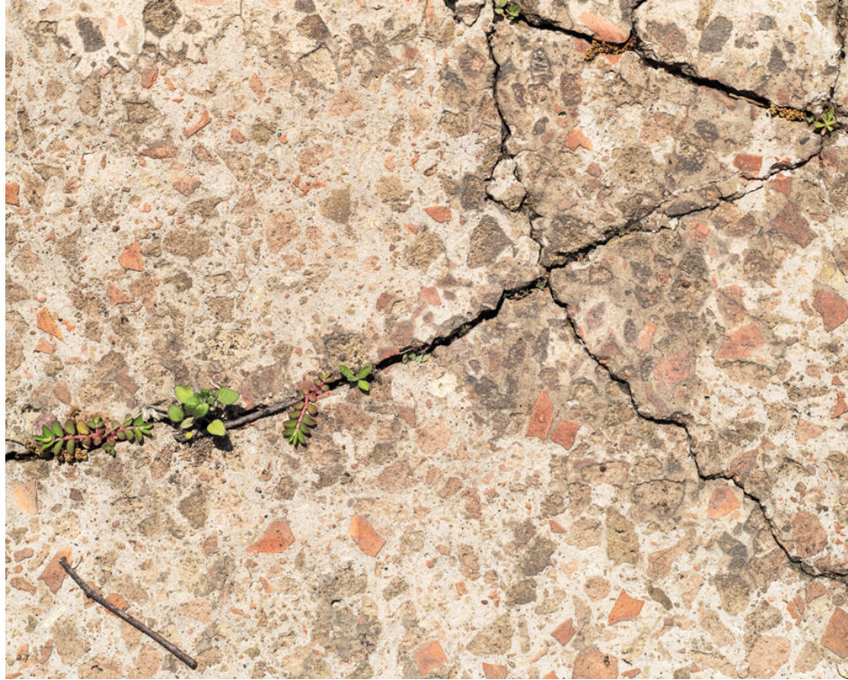
Figure 70: Detail of northern section of cocciopesto pavement of western cella, 2016 (author).
