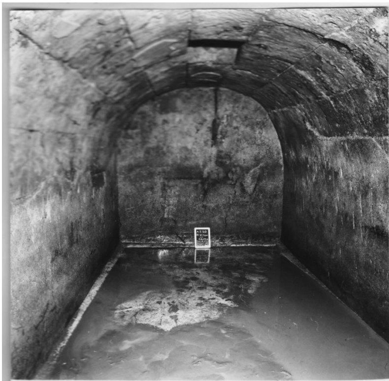
Figure 28: Central cistern, northern end, June 6, 1980 (ASRCM, S. Omobono, b. 31, 1, 4051.219).
