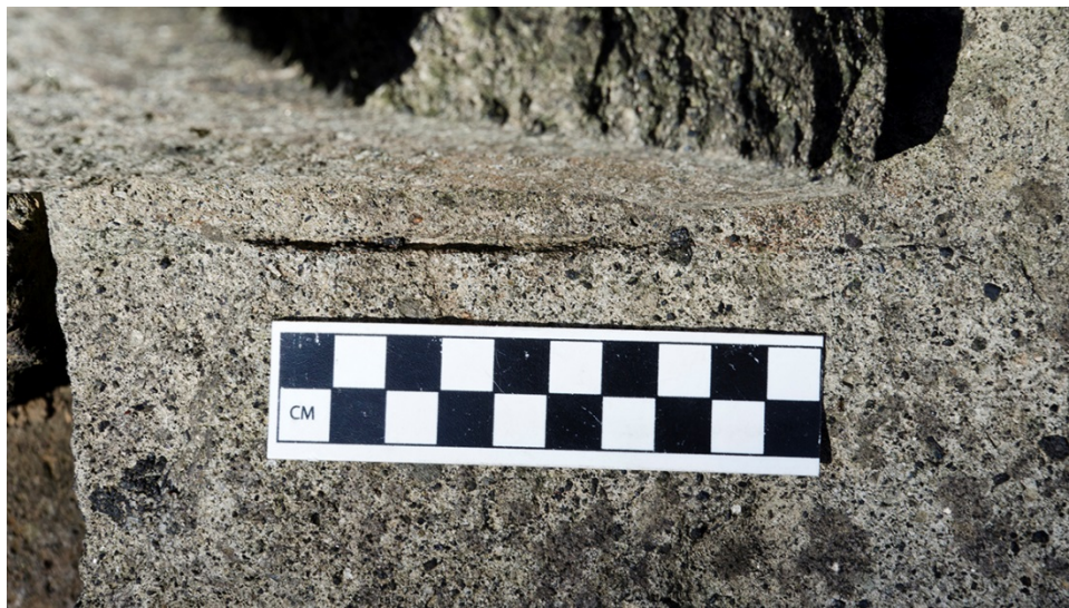
Figure 49: Incised setting line at southeastern corner of northern base-molding block of eastern altar (author).
