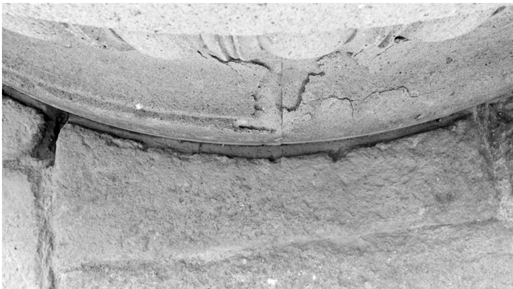
Figure 61: Gap between northern edge of circular monument and surface of Anio block pavement (author).
