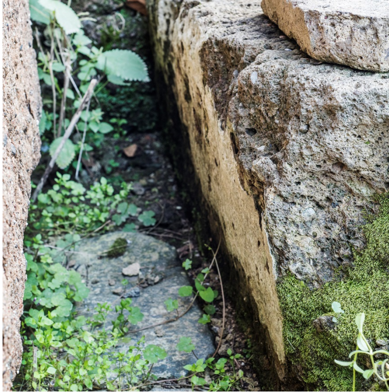
Figure 13: Plaster on exterior face of Tufo Giallo block of the “Taberna Republicana” (author).
