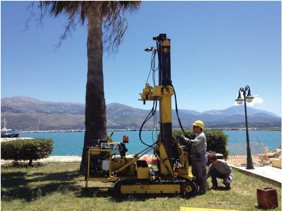
Figure 6.9: DPT Test Rig - Cephalonia, Greece
