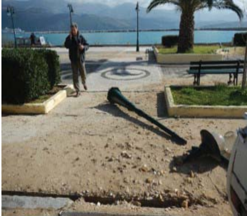
Figure 6.5: Observations of gravelly soil liquefaction at Lixouri Port ( Nikolaou et al. , 2014)
