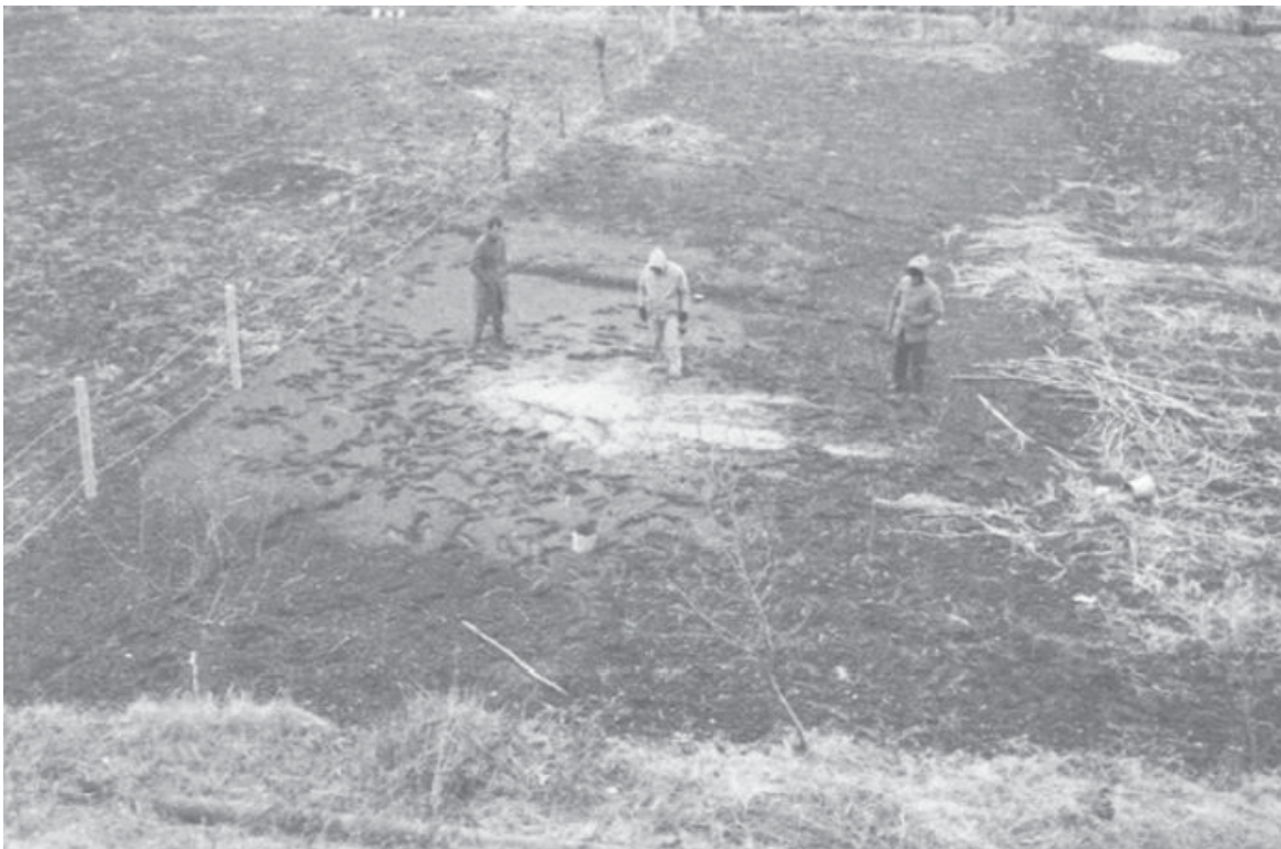
Figure 2.43: Sand boil observed near roadway embankment, 1988 Armenia earthquake ( Yegian et al., 1994 )
