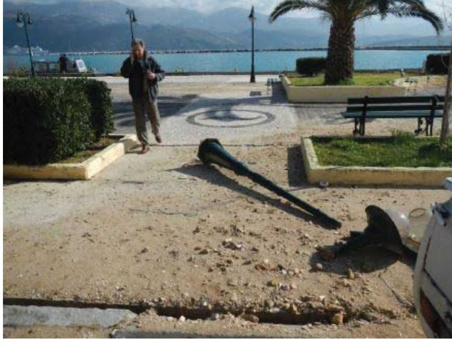
Figure 2.54: Observed gravelly soils ejected from the ground during liquefaction, 2014 Cephalonia earthquake ( Nikolaou et al. , 2014)
