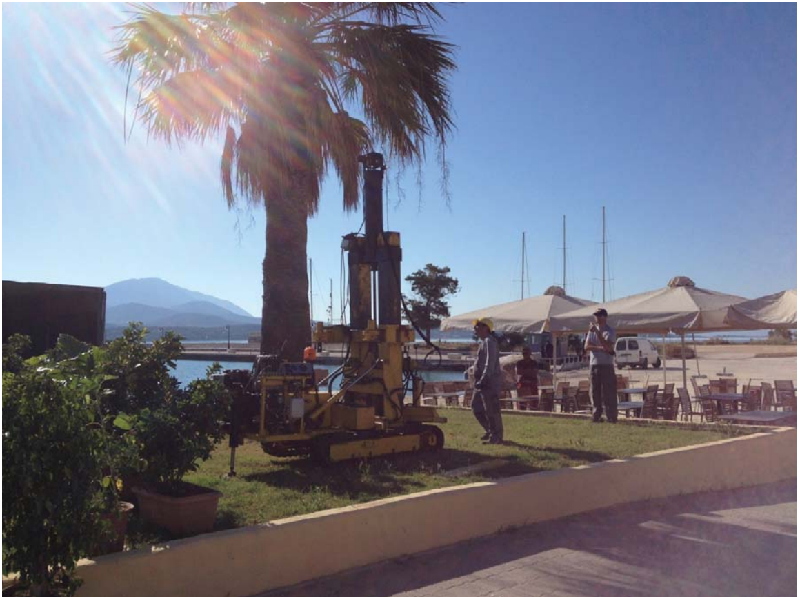
Figure 6.27: Setup of DPT at Location 1 in planter box
