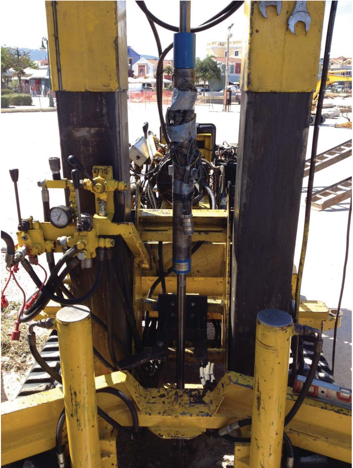
Figure 6.14: Instrumented rod placed in drill rig for energy measurement
