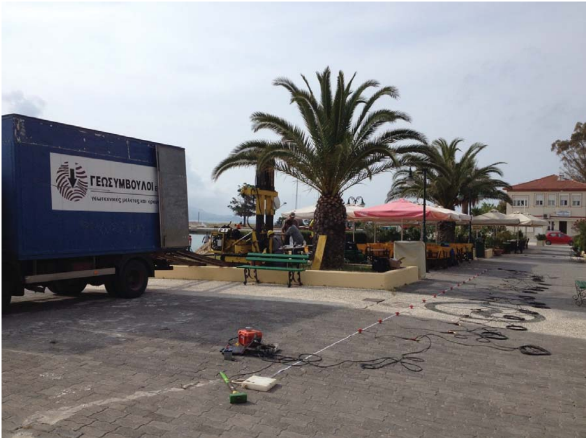
Figure 6.33: Setup of DPT and V_S Measurements at Location 3
