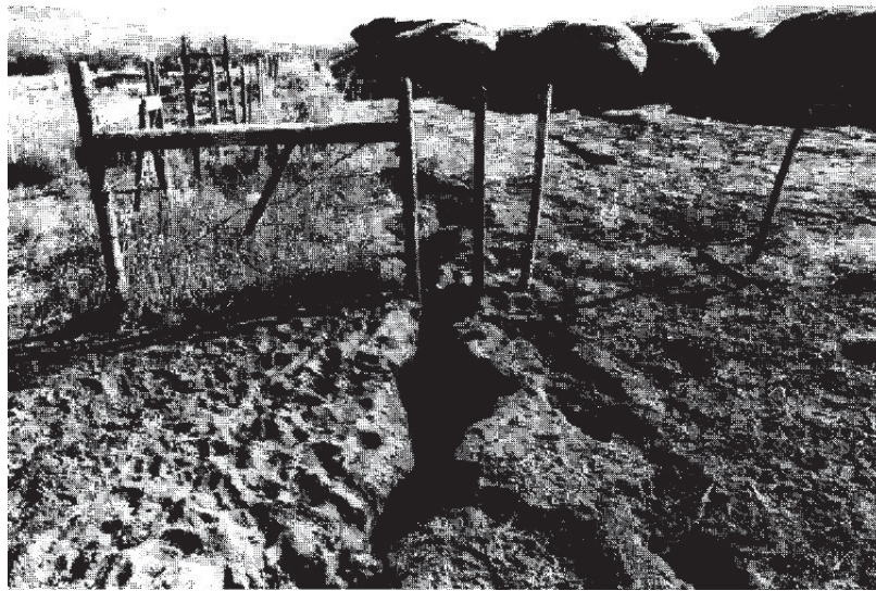
Figure 2.38: Ground fissure observed following the 1983 Borah Peak earthquake ( Youd et al., 1985 )
