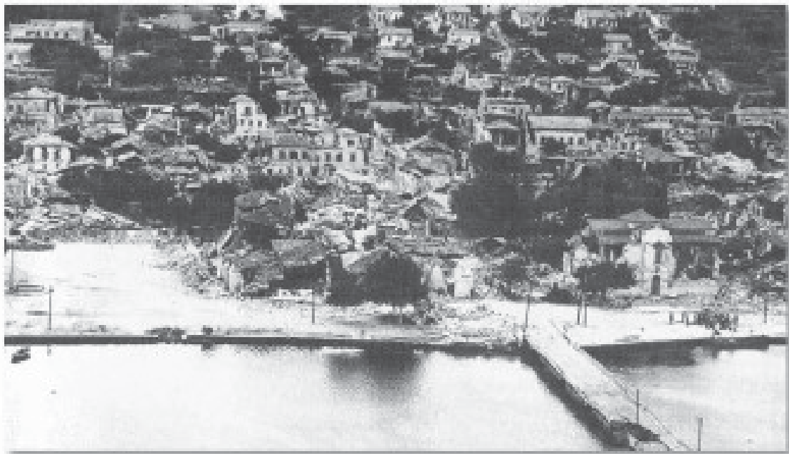
Figure 6.2: Damage observed in Argostoli during 1953 Earthquake (Nikolaou et al., 2014)
