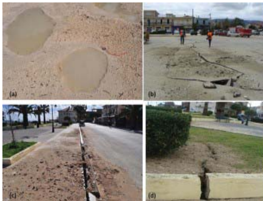
Figure 6.4: Observations of liquefaction at Lixouri Port ( Nikolaou et al. , 2014)
