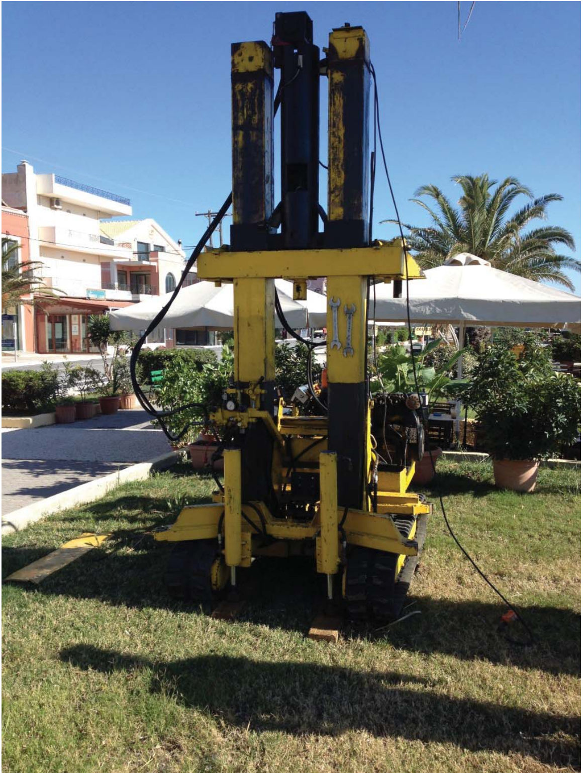
Figure 6.8: DPT Test Rig - Cephalonia, Greece
