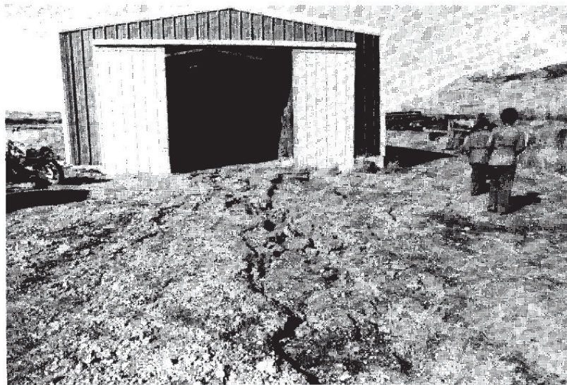
Figure 2.37: Ground fissure observed following the 1983 Borah Peak earthquake ( Youd et al. , 1985)
