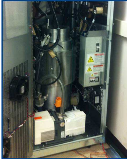
Figure 3.3: Flywheel module of MPEL test-bed.
