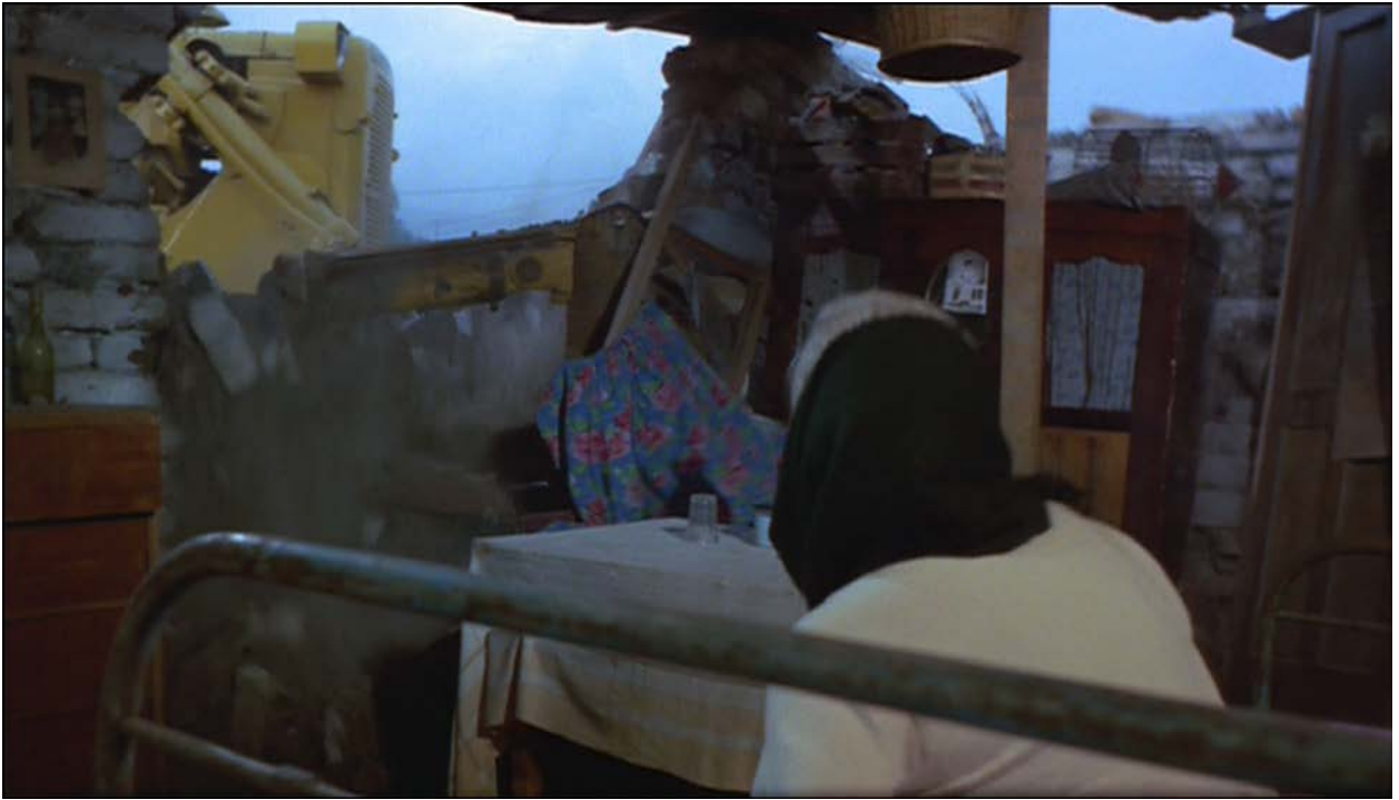
Image 2.4: A home is bulldozed, Tivoli .
