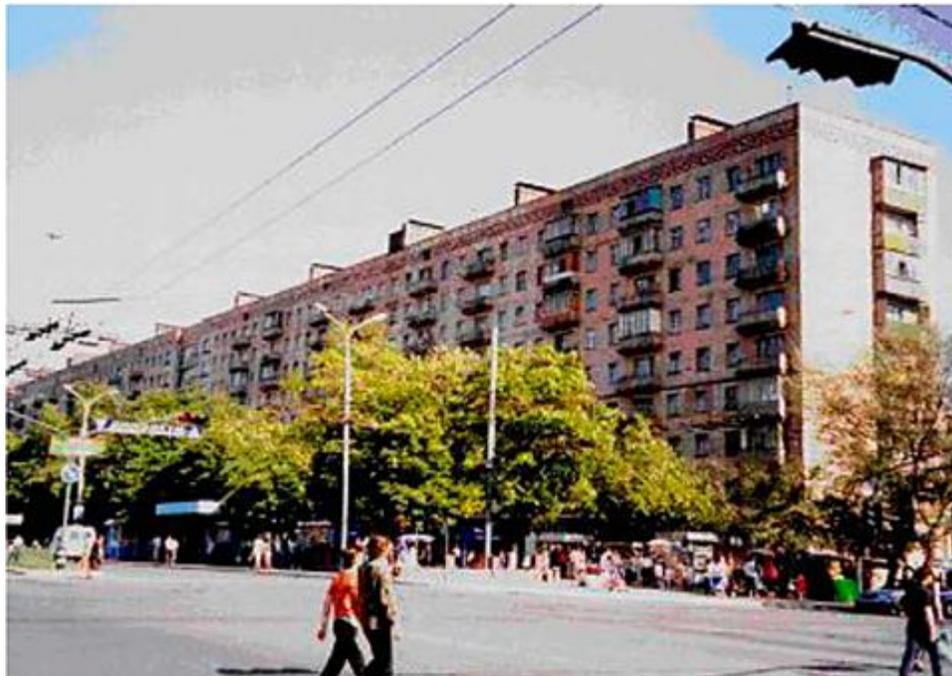
**Fig. 2.3:** Residential building made of alkali-activated slag concrete in Mariupol, Ukraine, 1960 [12]. The alkali-activation technology found various applications in the former Soviet Union.
