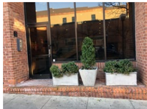
Figure 6: Planters occupy the ledge next to the 101 W. Liberty entrance. The edge of the brick where the street slopes downward offers opportunity for sitting, despite the planters.
