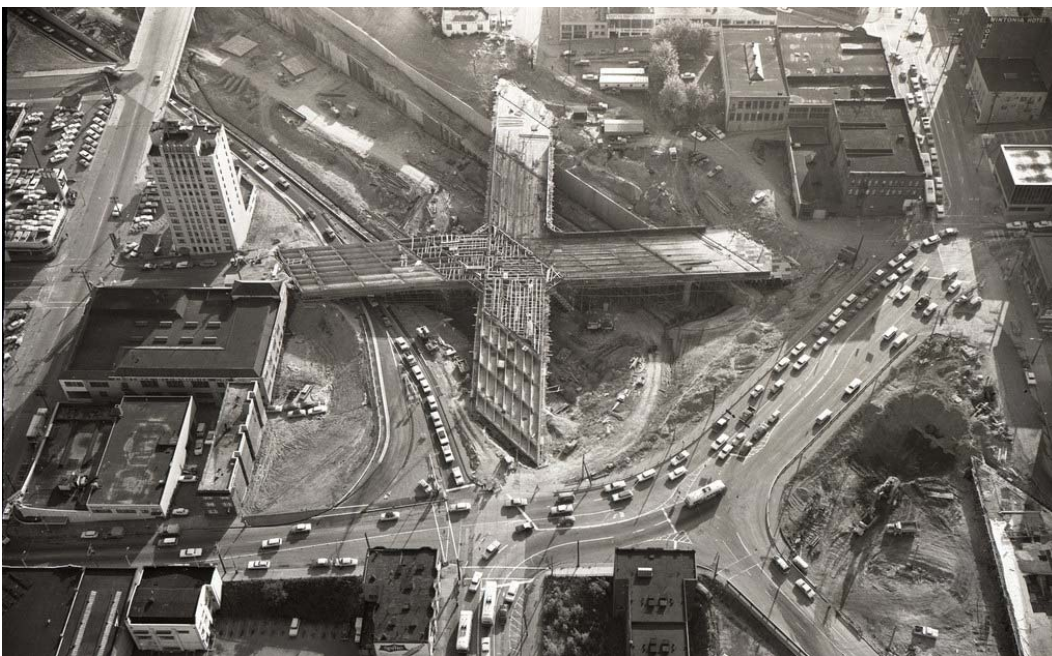
Figure 4.17. Pine and Boren intersection during I-5 construction, 1965.
