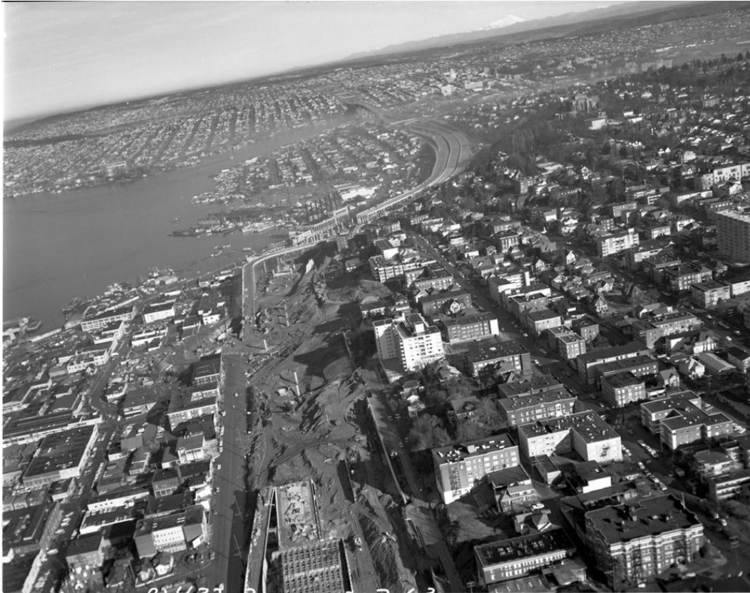
Figure 4.16. I-5 construction through central Seattle looking north from Downtown, 1963.
