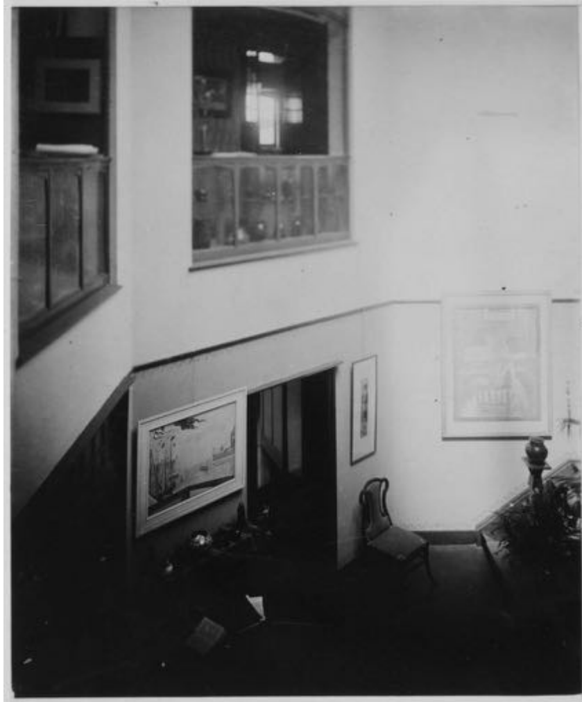
Figure 111 View of the Living Room at Bloemenwerf with Seurat's Grande Isle and van Rysselberghe's Maria Sèthe at the Harmonium, c. 1894. Archives d'Architecture Moderne, Ixelles.
