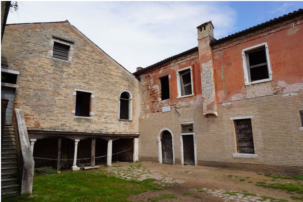
Figure 3.33: Prior's house and courtyard
