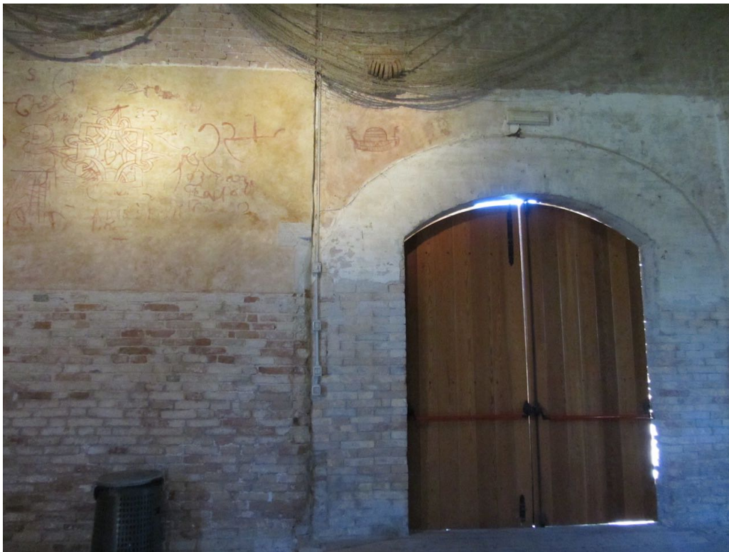
Figure 3.39: Interior view of tezon grande with graffiti above and beside door
