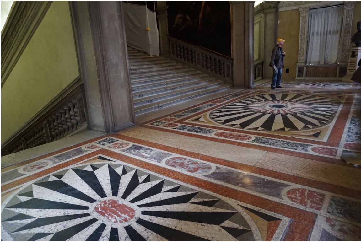
Figure 5.7: Stone inlay on the landing of the grand stairway in the Scuola Grande di San Rocco
