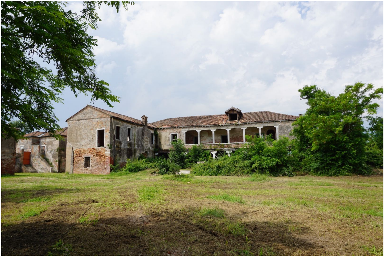
Figure 3.13: Cloisters at the Lazzaretto Vecchio
