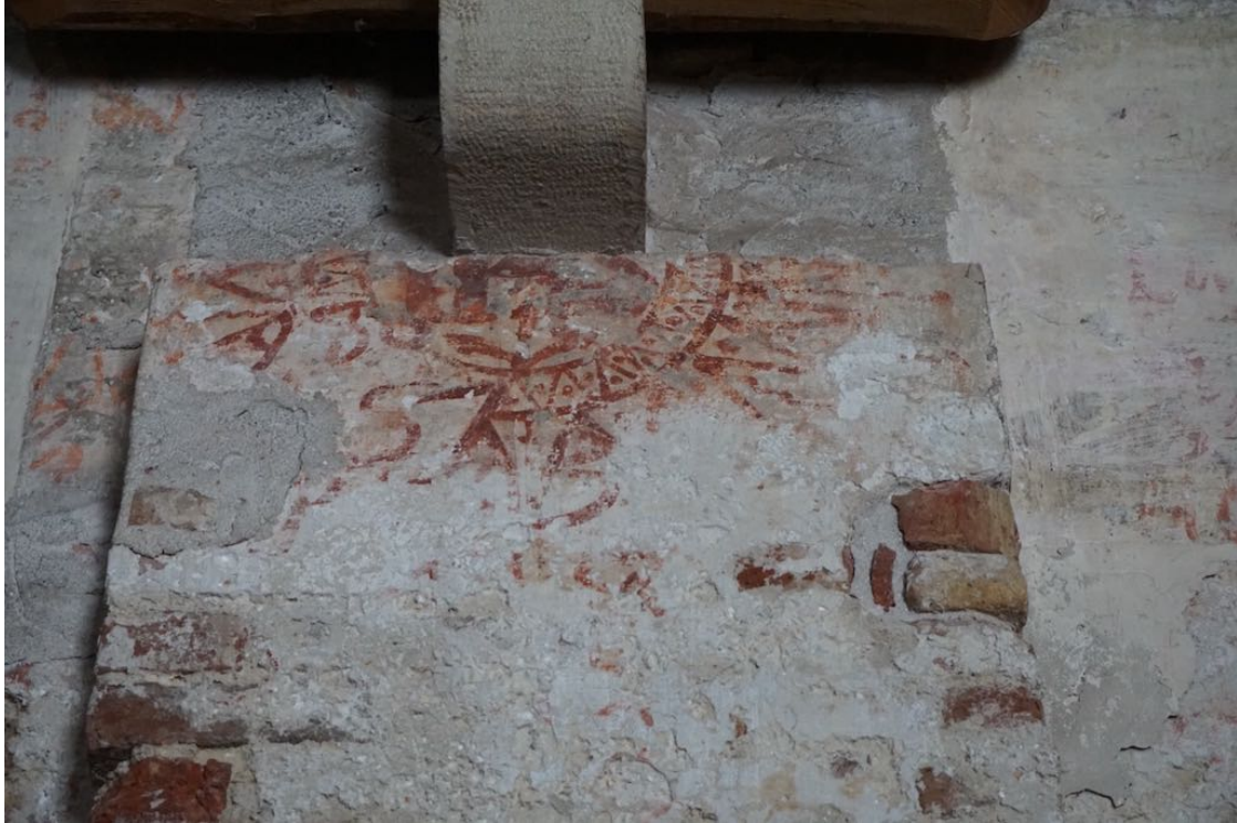
Figure 3.44: Graffito damaged by structural additions at the Lazzaretto Vecchio
