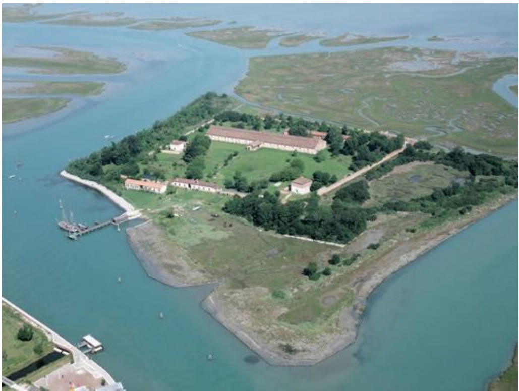
Figure 3.4: Lazzaretto Nuovo, aerial view
