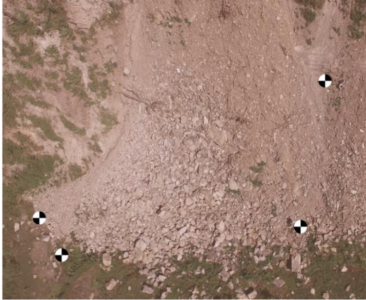
Figure 3-14: GCPs placed at the landslide toe
