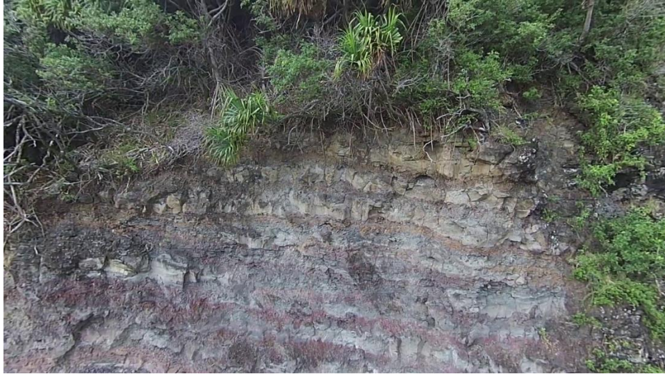
Figure 3-17: UAV-collected image at top of landslide scarp showing alternating stratigraphy
