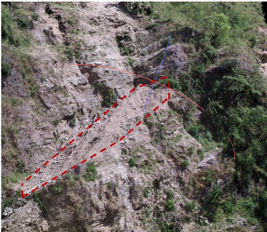
Figure 3-28: Structurally-controlled, wedge failure observed about 50 m upslope
