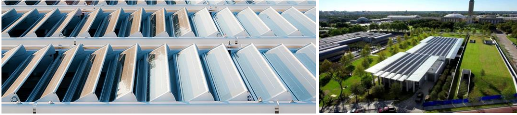
Figure 4.10. Exterior blinds installed on the skylights of the Kimbel Museum extension (Piano, n.d.)
