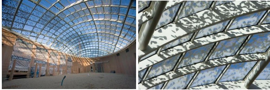
Figure 4.14. Interior of the main enclosure in the New Elephant House (a); detail of the frit pattern (b) (Foster, n.d.)
