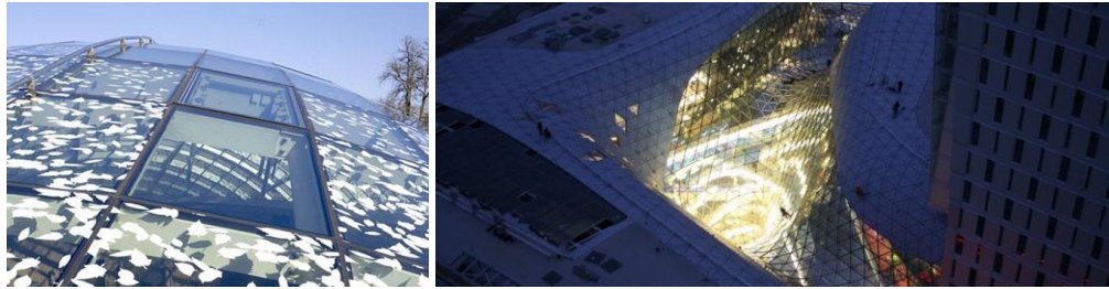
Figure 4.17. Alternating fritted and transparent panels at the New Elephant House, alternating opaque (a); transparent panels at the MyZeil Shopping Mall (b)
