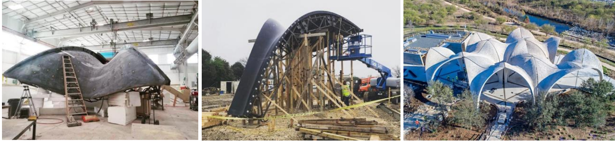
Figure 3.22. Concrete shell in Confluence Park, San Antonio, Texas
