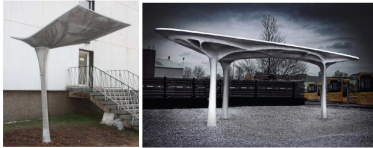
Figure 3.20. Shell with a wiremesh (a) (Eisenbach, Vasudevan, Grohmann, Bollinger, & Hauser, 2014); a shell manufactured with CNC milled formwork (b) (Dombernowsky & Søndergaard, 2012)
