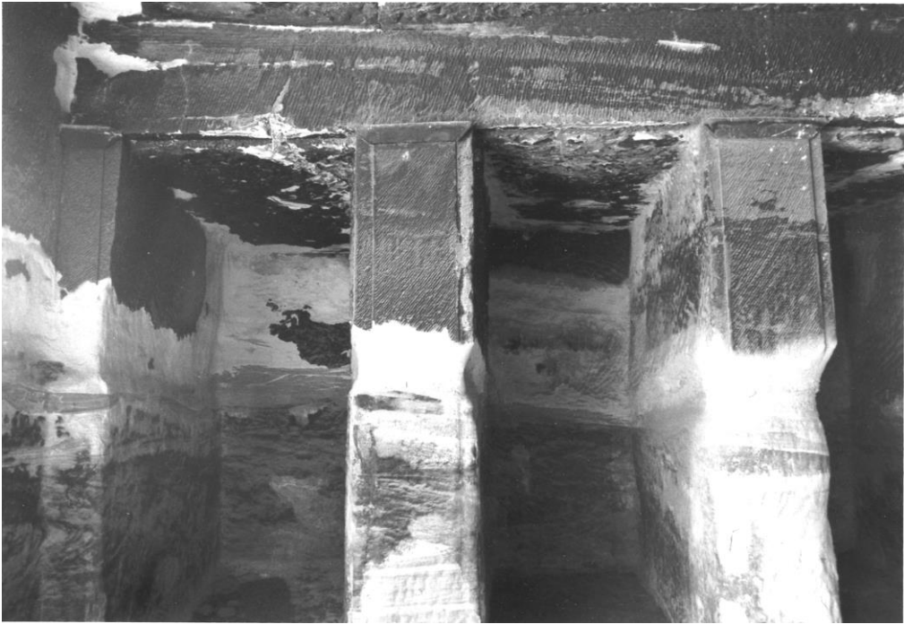
c. Detail of eastern wall (2-9-1997)
