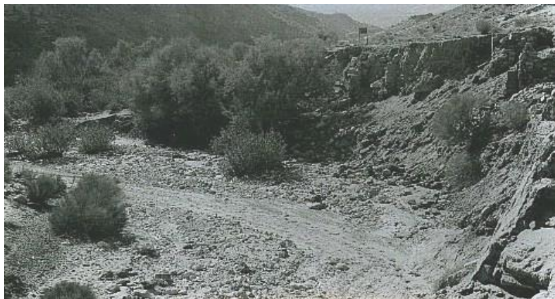
c. Fallen walls in Wādi Sabrah / South-west of Petra (13-2-1993)
