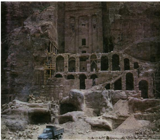
b. Staircase under restoration (s.1978)
