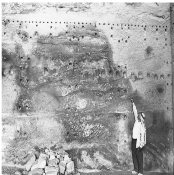
c. Detail of lower part of south wall (2-15-1997)
