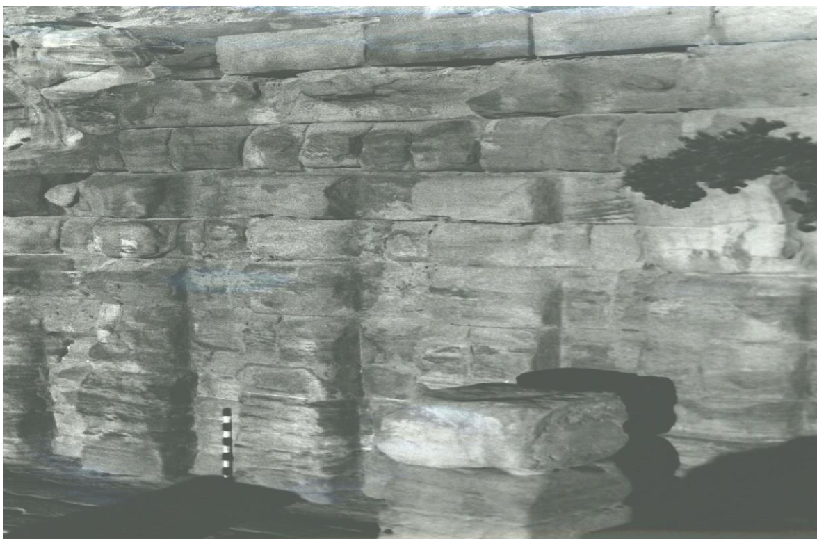
b. From south looking north (11-9-1993)
