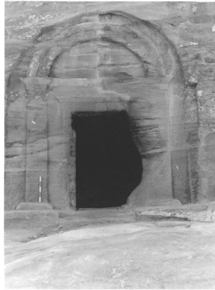
b. Finished façade (Br. 578) (2-11-2000)
