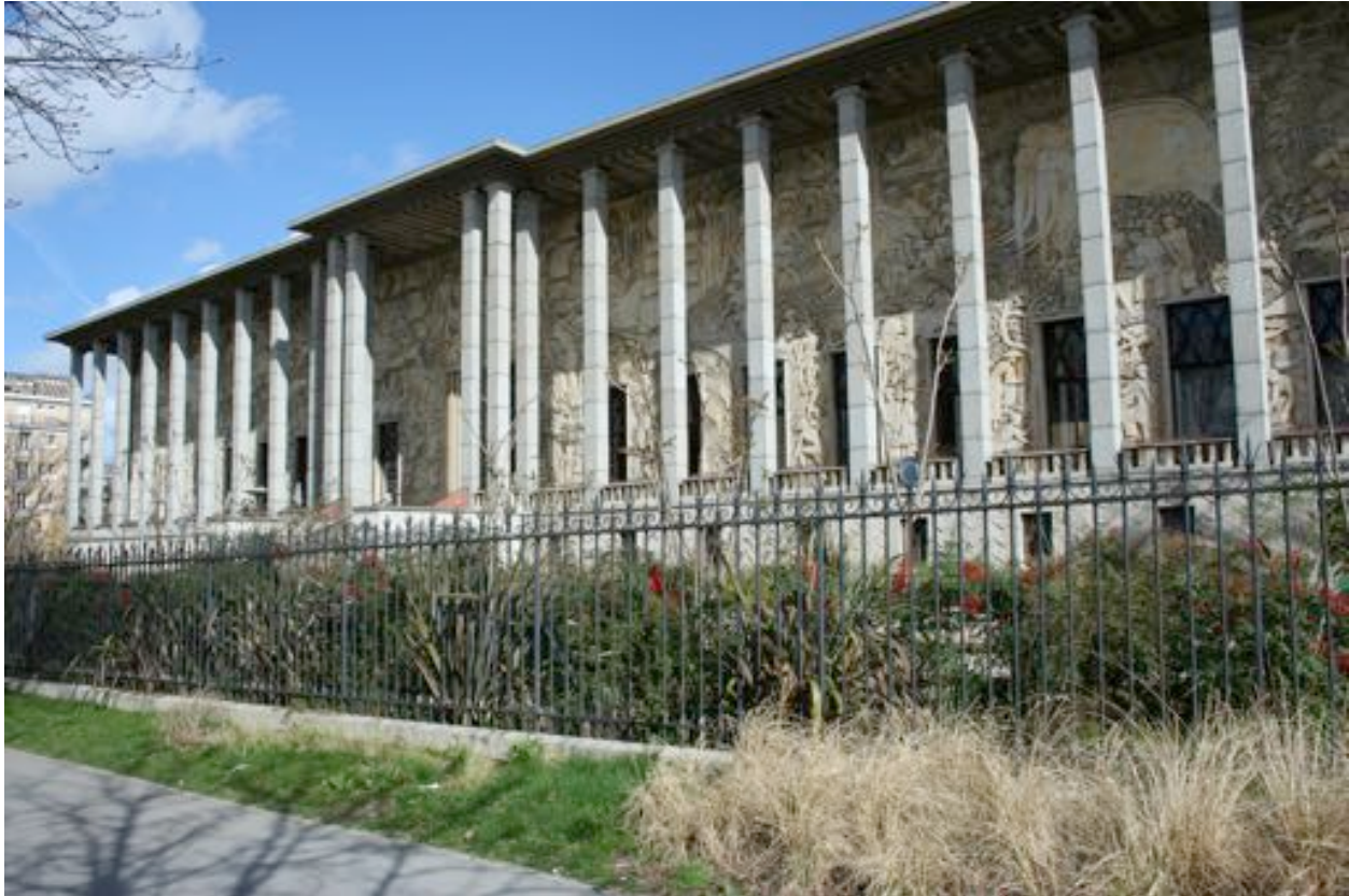
Figure 3 Facade of the MNHI. Photo courtesy of author.
