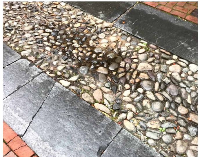
Images 58 (Top), 59 (Bottom), 60 (Right): Also a tourist attracting, revealing many ideas of the built environment during colonial times. (Source: Authors)
