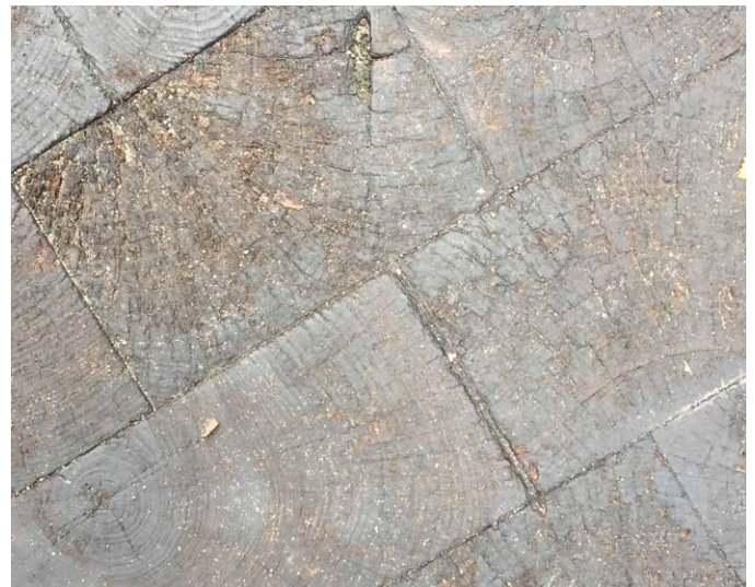
Images 41 (Top), 42 (Bottom), 43 (Right): As seen from the images above, the wooden pavers form the same aesthetic as brick pavers. The slight growth of moss is seen in the alley. The experience was more comfortable as compared to conventional alley pavers, through its historic appeal and retaining of air moisture. (Source: Authors)
