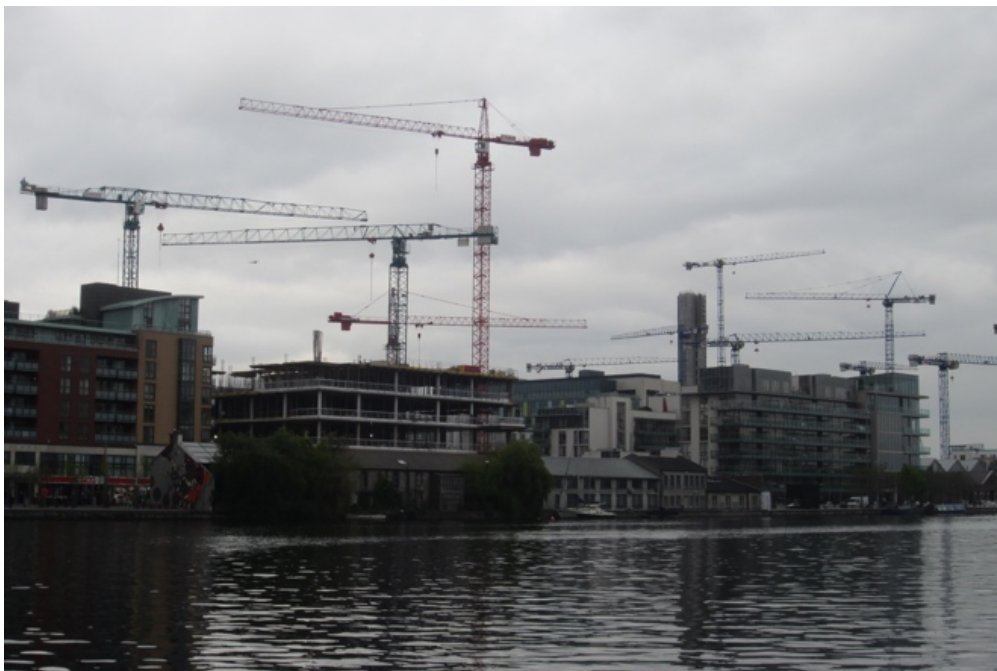
Figure 7: Construction of the Silicon Docks south of the Liffey river
