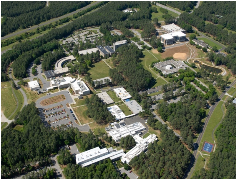
Figure 33: Aerial view of Research Triangle Park
