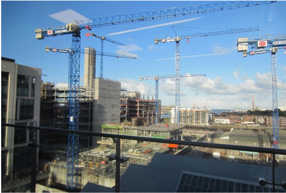
Figure 6: Construction of the Silicon Docks south of the Liffey river
