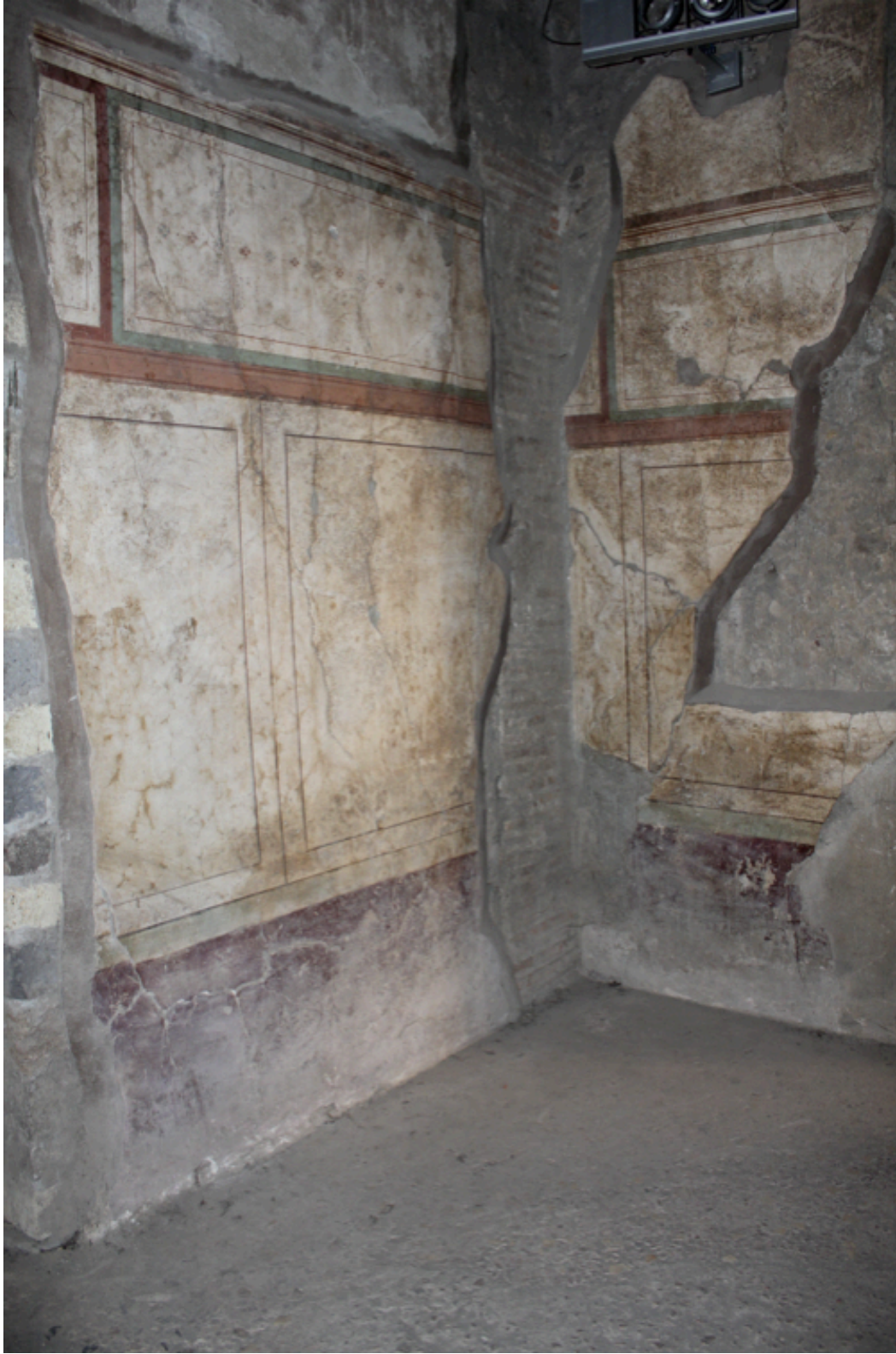
Figure 28. Villa A, Oplontis. Room 10b looking northwest.
