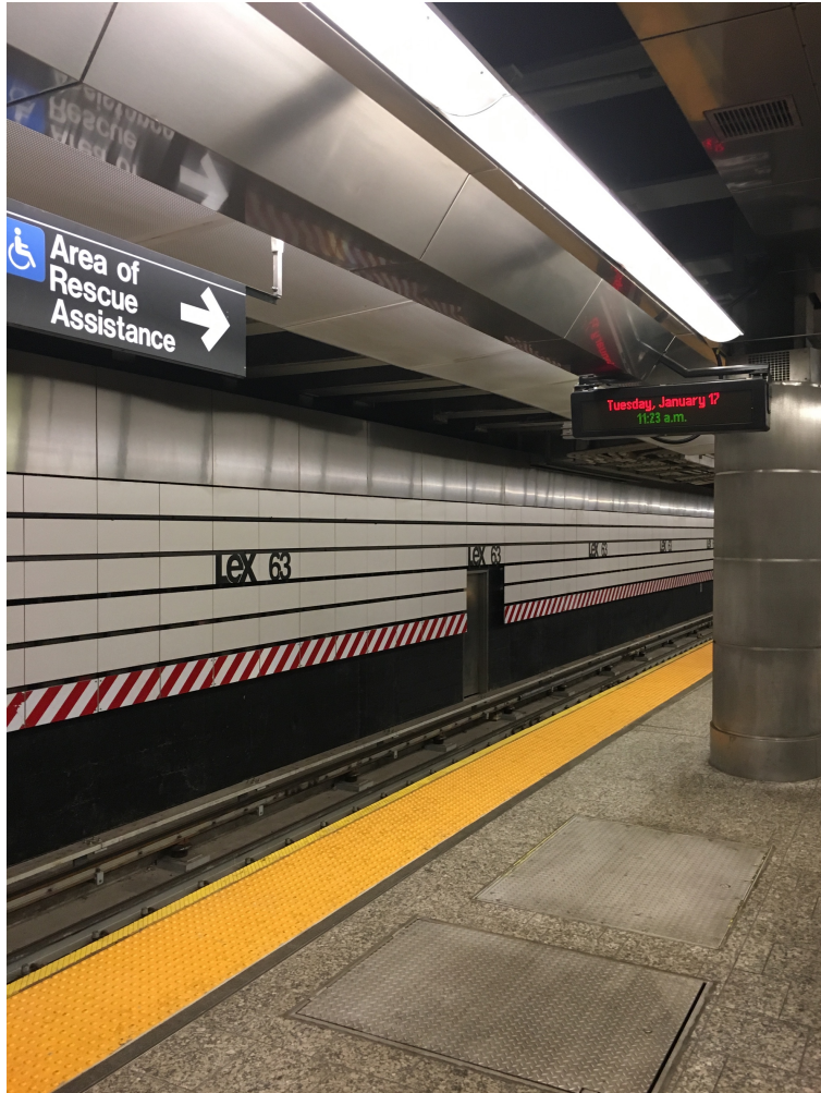
Figure 39. Subway platform at Lexington Avenue/63rd Street.
