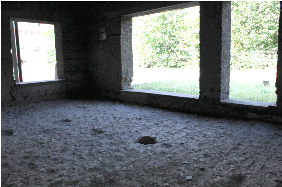
Figure 14. Villa A, Oplontis. Diaeta 78, view towards northwest.
