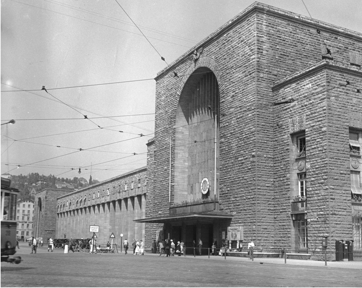
Figure 1.15 Paul Bonatz and Friedrich Eugen Scholer, Stuttgart Main Station, Stuttgart, Germany, 1911-27. Photograph by Norman Charles Westwood. Copyright Bryan & Norman Westwood / RIBA Collections.
