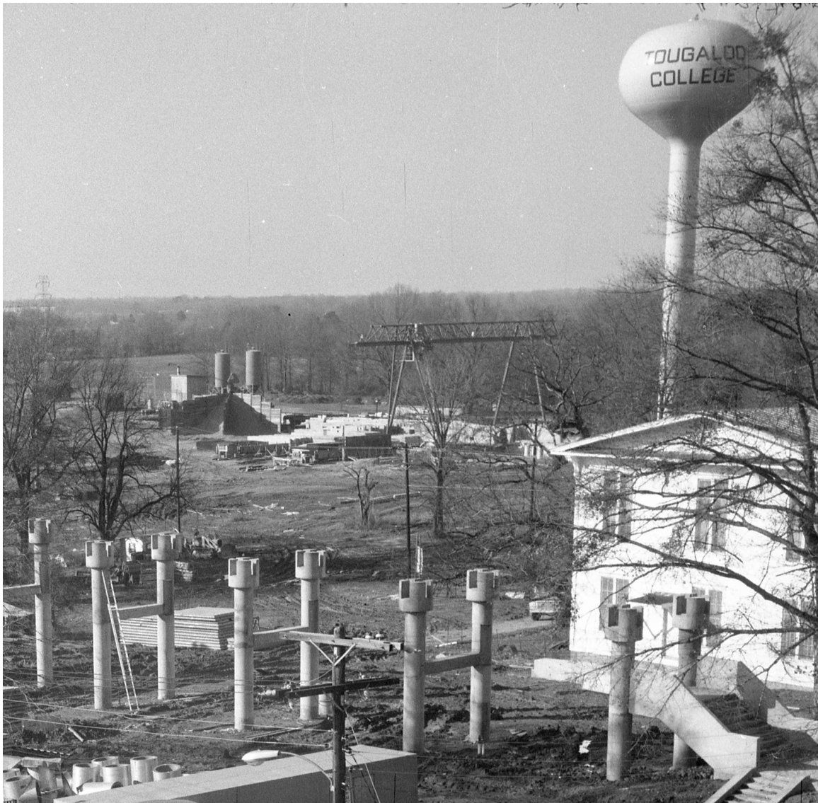
Figure 2.13 Detail of Tougaloo College construction photograph showing Burnett precasting plant set up on campus, next to the water tower, to produce panels for dormitory construction. Box 5, GBA records, BHL.
