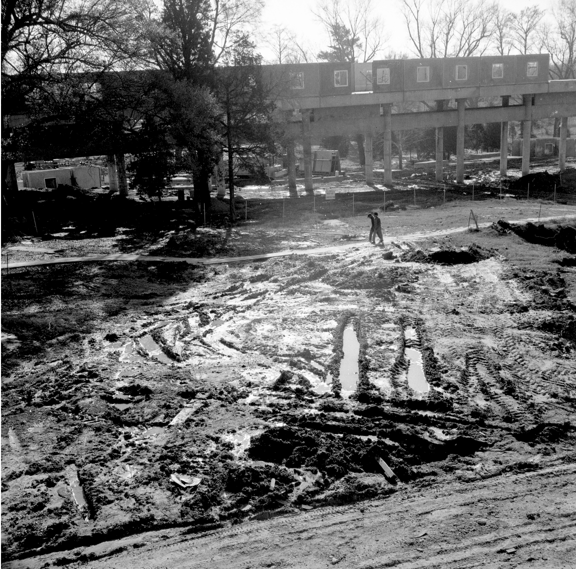
Figure 2.06 Tougaloo College construction photograph showing muddy Yazoo clay soil on library construction site, with dormitory in background. Box 5, GBA records, BHL.
