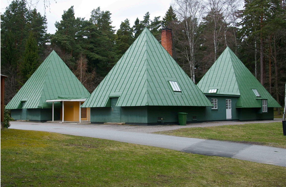
Figure 1.28 Erik Gunnar Asplund, Staff Building, Woodland Cemetery, Stockholm, Sweden, 1923. Photograph by Arild Vågen courtesy Wikimedia Commons. https://commons.wikimedia.org/wiki/File:Tallum_Pavilion_2012b.jpg (Accessed 3 April 2017).
