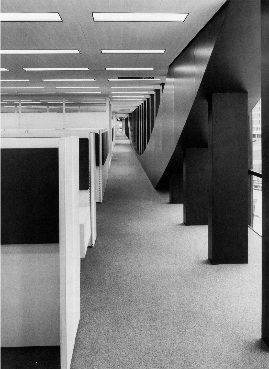
Figure 3.47 Interior of purchasing department on floor 2, FRBM office tower, with General Fireproofing workstations and demountable partitions at left, and bottom of catenary suspension structure at right. Photograph by Balthazar Korab. From: Birkerts and Schwartz, 109.
