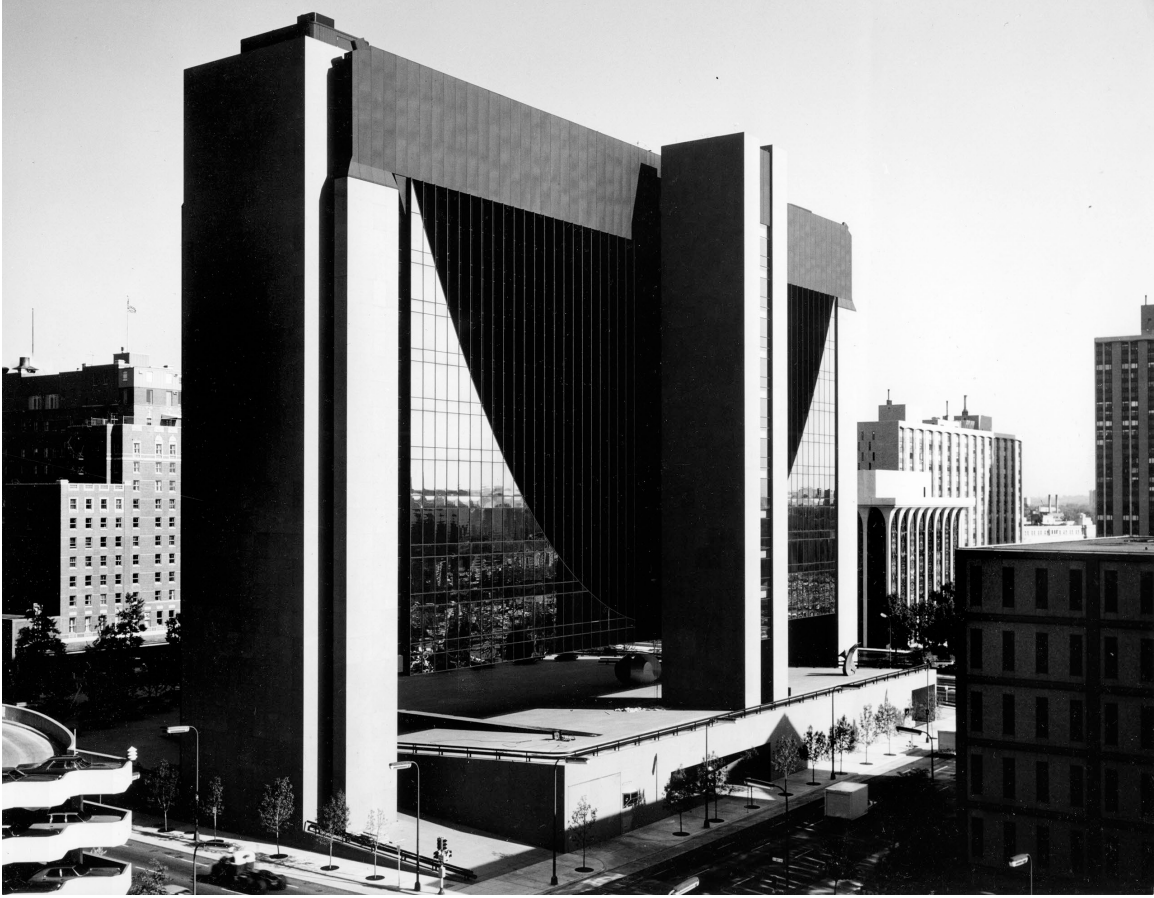
Figure 3.50 Oblique view, northeast facade of FRBM, ca. 1970s. Black and white print, 8 x 10 inches. Photograph by Balthazar Korab. Box 13, GBP, BHL.
