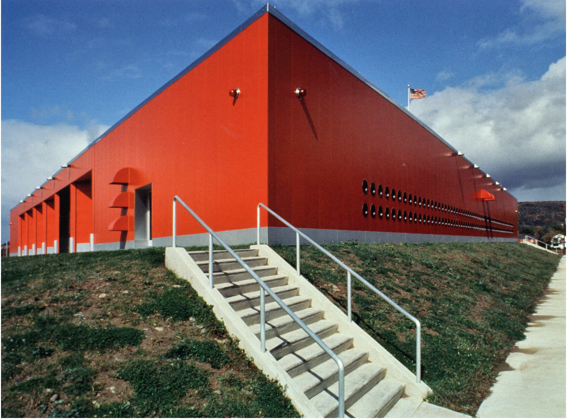
Figure 4.16 GBA, Corning Fire Station, Photograph by Paul Chu Lin. From: Birkerts and Schwartz, 65.
