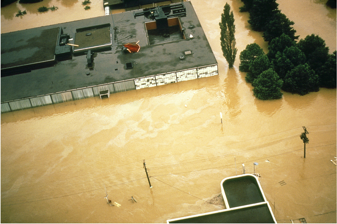
Figure 4.06 Corning Glass Center engulfed by floodwaters, June 23, 1972. Courtesy Corning Museum of Glass. From: https://www.cmog.org/article/flood-1972 (Accessed October 13, 2018).
