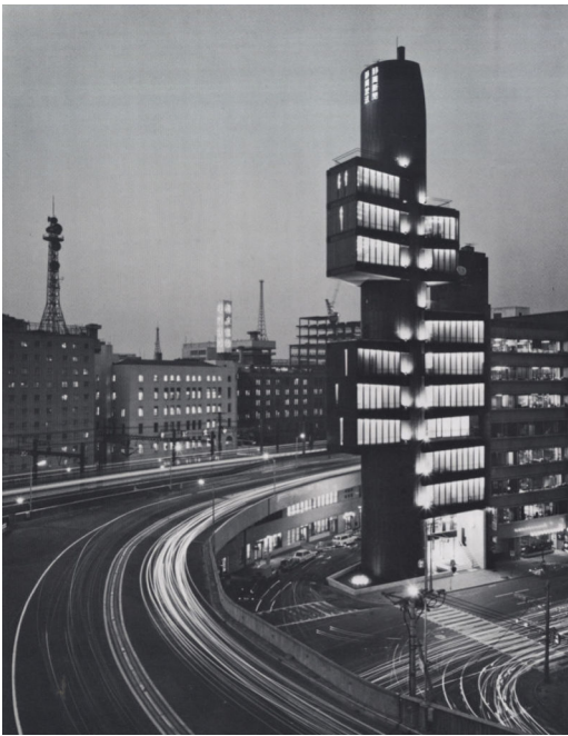
Figure 4.26 Kenzo Tange & URTEC, Shizuoka Press and Broadcasting Centre, Tokyo, Japan, completed 1967.
