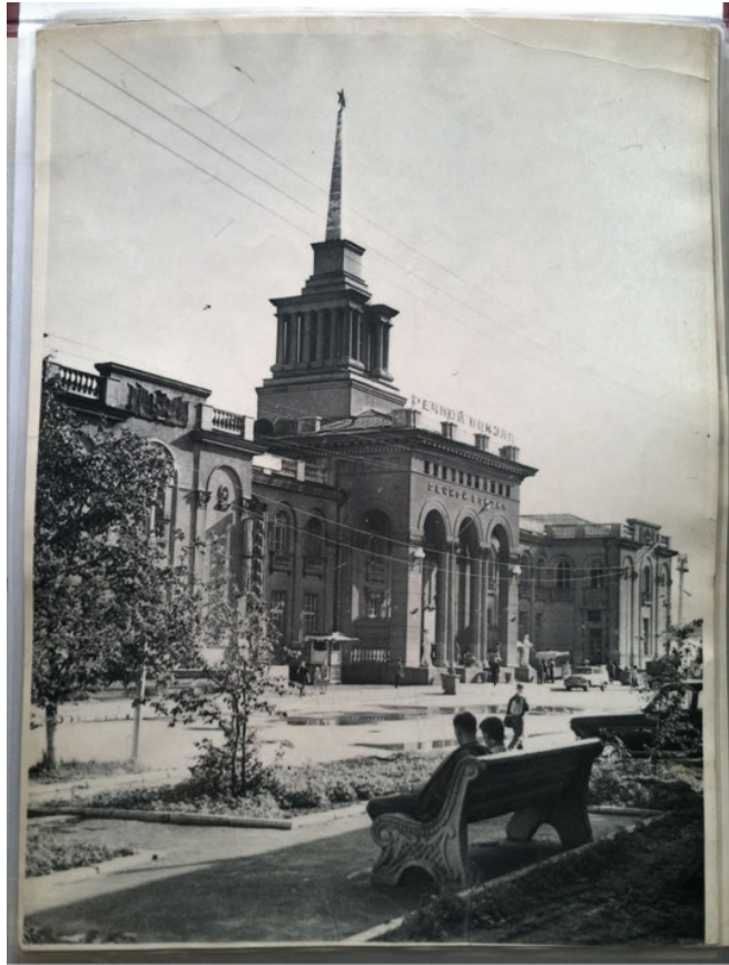
Figure 5.8 Photograph of Krasnoyarsk River Station ( Rechnoi Vokzal ), completed in 1952, showing street amenities ( blagoustroistvo ) in foreground 84
