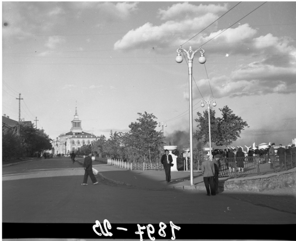
Figure 5.17 Photograph of Krasnoyarsk embankment near River Station, June 1955 93
