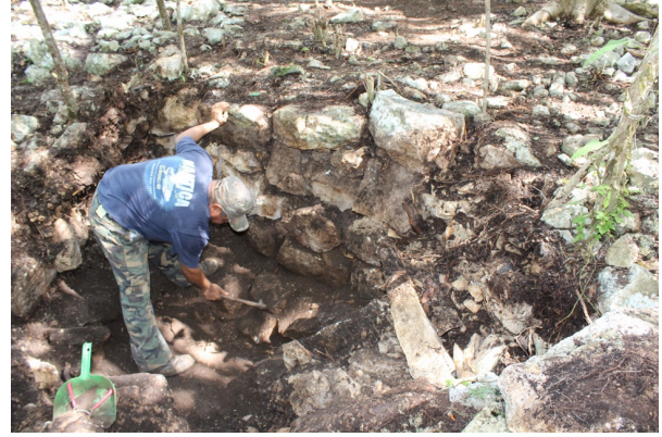
Figure 6.19 Excavating earlier basal platform wall on the south side of the Jach Group
