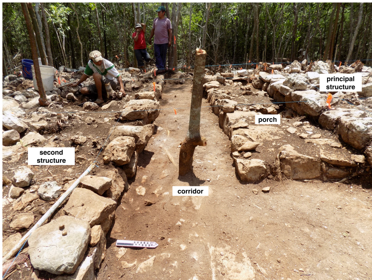
Figure 6.97 View of the Chamal Group superstructures, showing the elements of the second phase of construction
